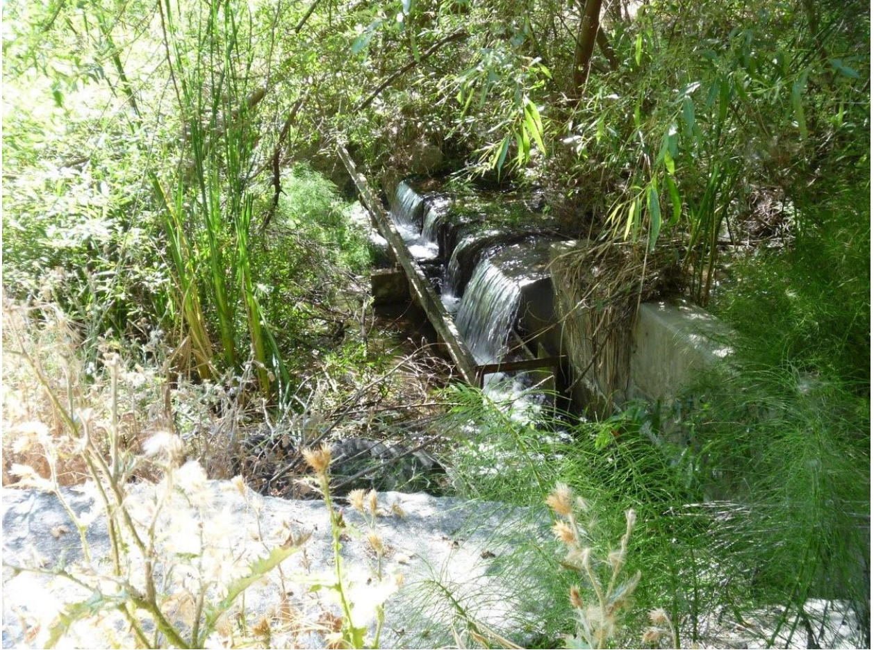
Pond 22 in-stream concrete retention dam
