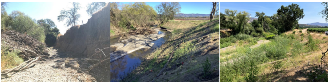
Figure 1: Group D - Site 4B of the Napa River Restoration Oakville to Oak Knoll Project showing steep eroding bank in the pre-project condition in September 2020 (left most photo), post-construction conditions with laid back banks and a floodplain secondary channel in April 2022 (middle photo), and native riparian and biotechnical vegetation establishment in July 2023 (right most photo).
