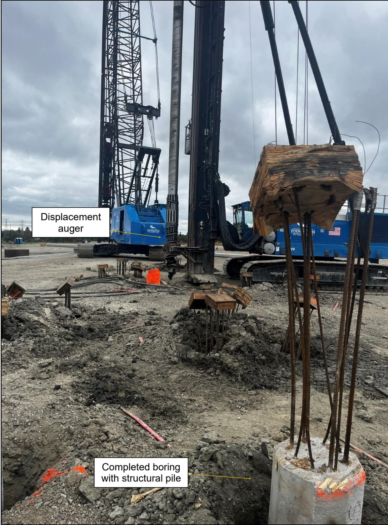
Figure 2. Construction site with displacement auger drill and borings.
