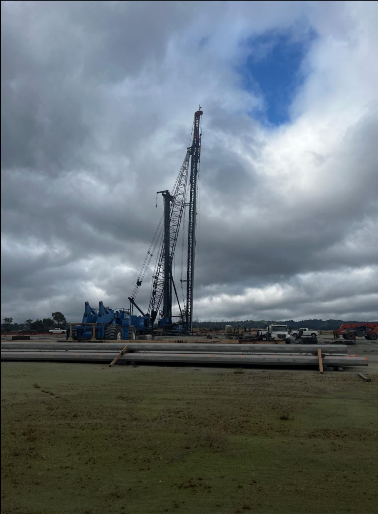
Figure 1. Structural piles in the foreground and pile-driving apparatus in background.
