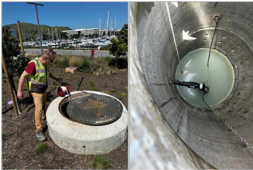
Figure 2: Exterior of the newly installed concrete sump basin (left) and interior showing the pump installed to divert lightweight cellular concrete related discharges to the sanitary sewer (April 2025).
