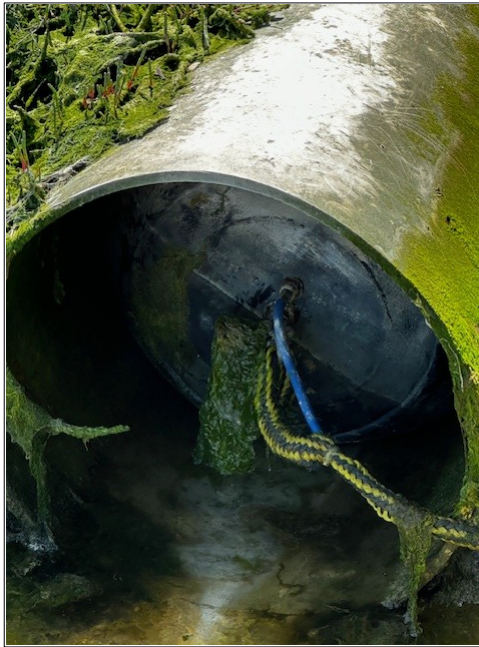
Figure 3: Inflatable bladder inside one of the outfalls (April 2025).
