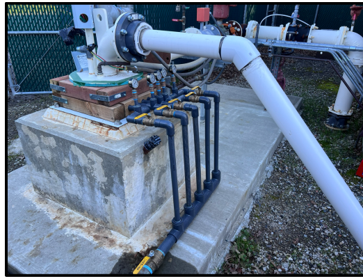
Figure 2: Verano Aquifer Storage and Recovery wellhead, showing injection manifold
