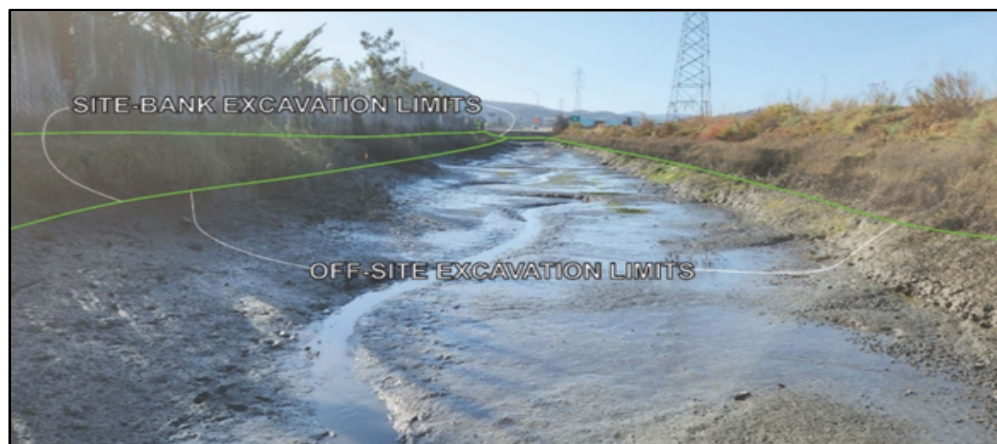
Figure 2: Offsite Ditch Prior to Remediation
