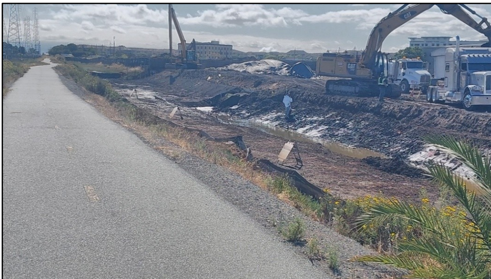
Figure 5: Offsite Ditch Sediment Remediation in Progress
