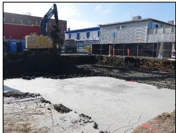
Figure 3: Excavation backfilled with cement slurry
