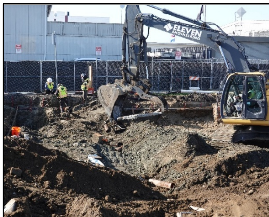
Figure 2: Removal of pipeline infrastructure
