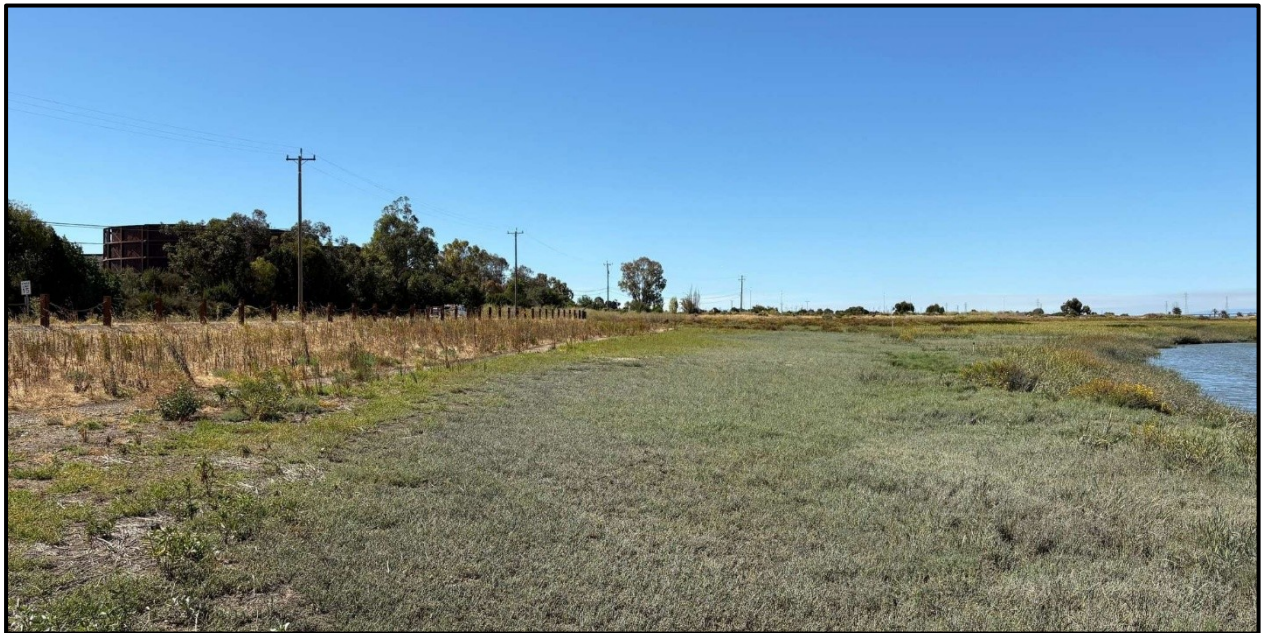
Photo 2: Horizontal levee slope with the improved public access trail to the left and Harbor Marsh to the right.
