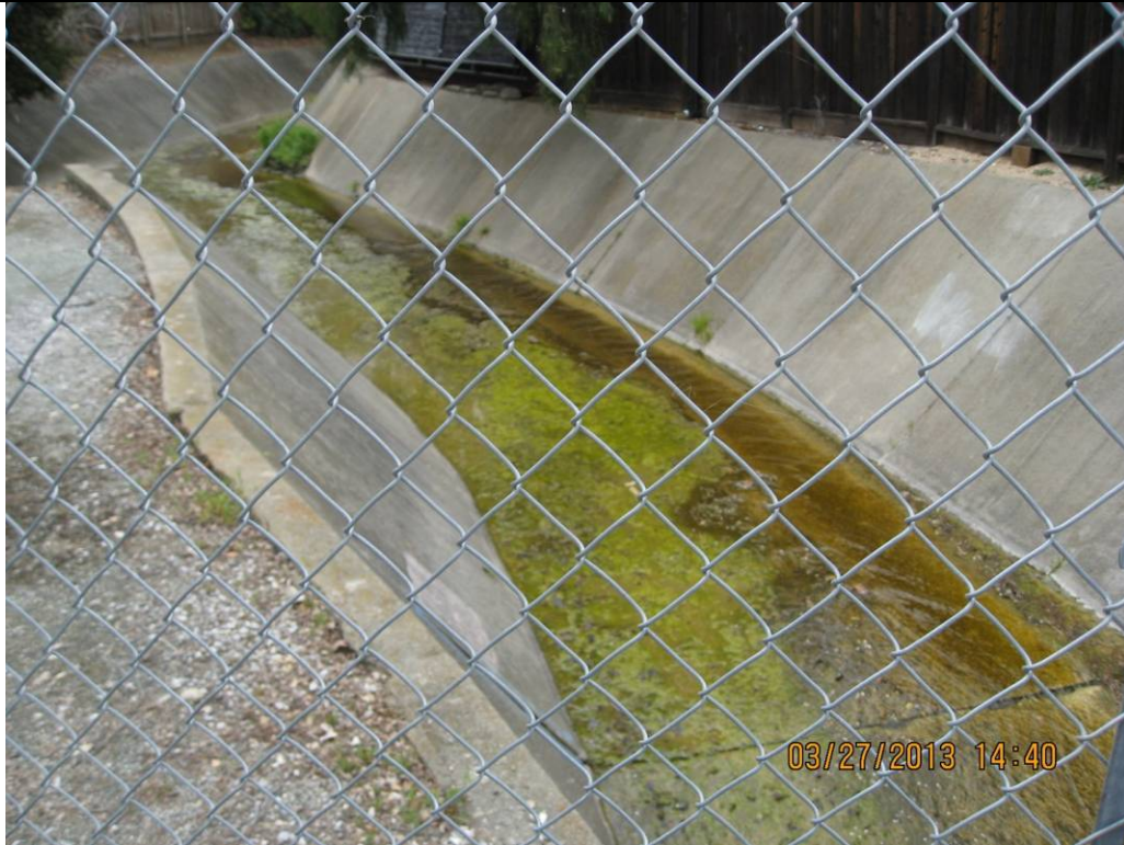
Hale Creek crossing at Mountain View Ave. (facing Northeast/downstream)
