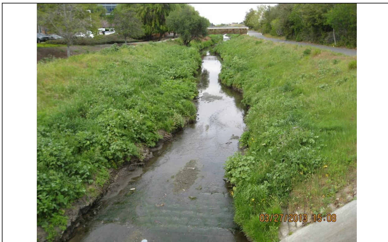
Permanente Creek crossing at Charleston Rd. (facing North/downstream)
