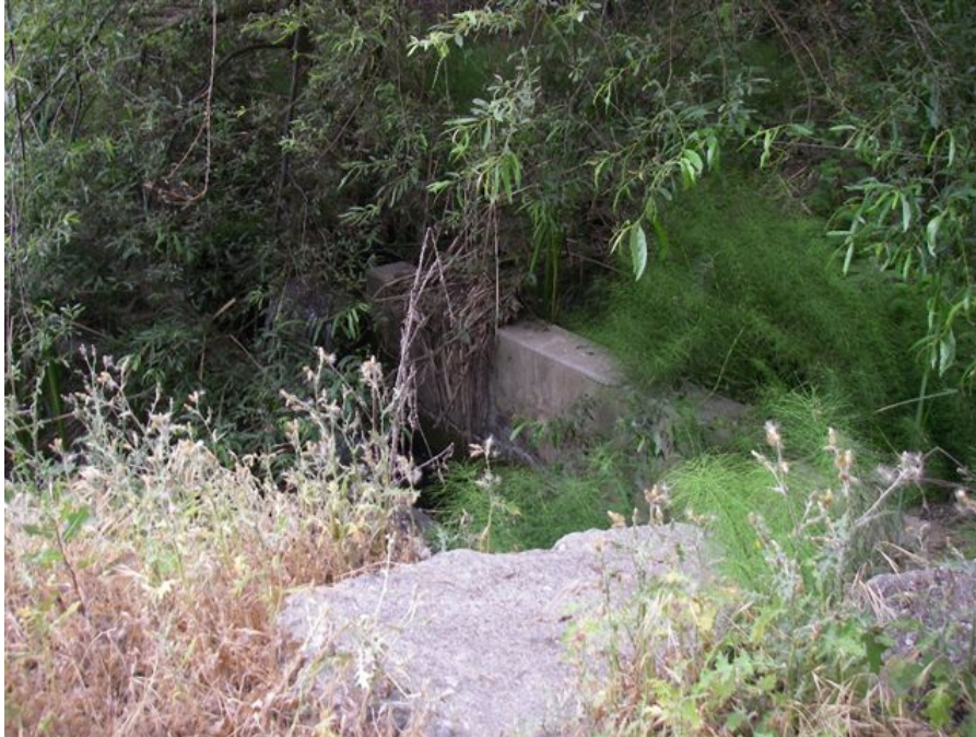
Photograph 7: Downstream terminus of Pond 22 at concrete weir
