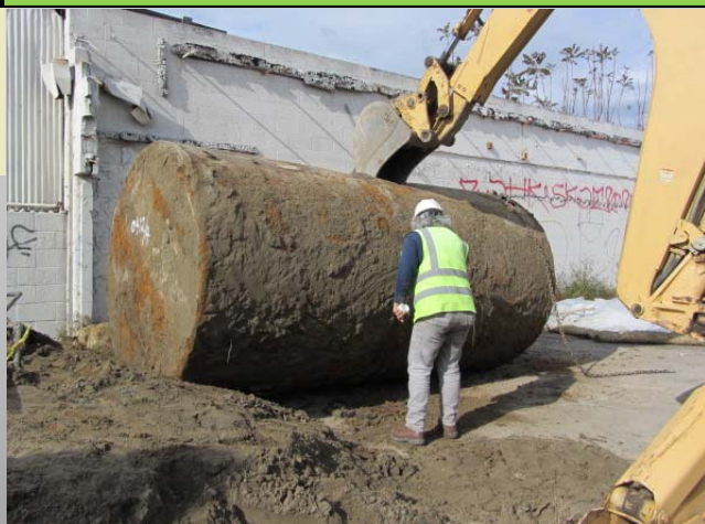
Photo 1: Excavation of 1000-gallon waste oil UST
