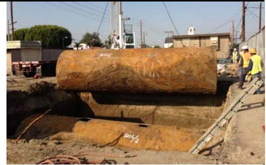
Photo 2: Removal of three 10,000-gallon USTs
