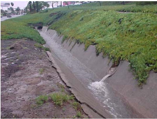
Arches Bioswale (pre-construction)
