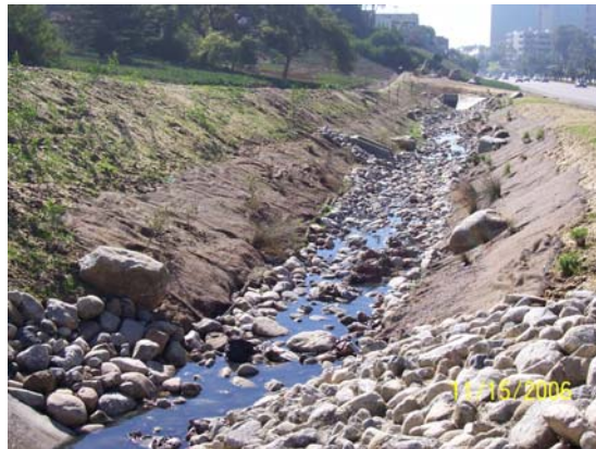
Arches Bioswale (post-construction)
