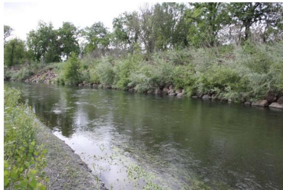
**Figure 2:** This photo was taken after completion of a bioengineered bank stabilization project on the Russian River at Stuhlmuller Vineyards.
