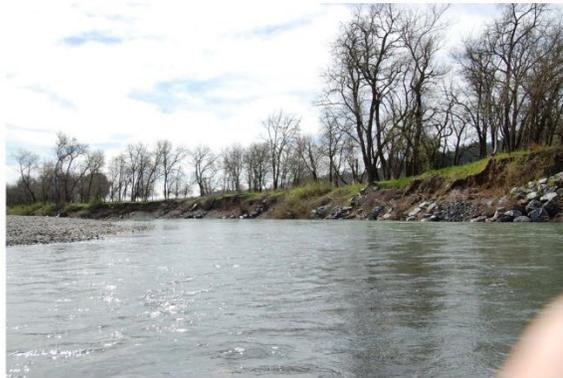
**Figure 3:** This photo is of the same stretch of project following the first high velocity flow event that the project experienced. It is clearly seen here that all the vegetation was removed during that high velocity event and the bank was further degraded.
