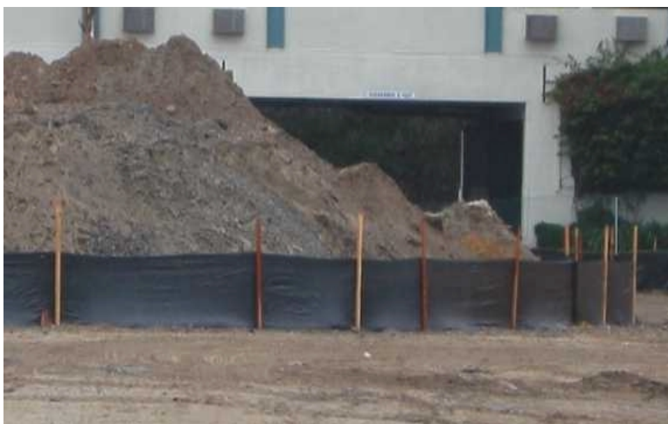
Silt fence used for stockpile perimeter control.
