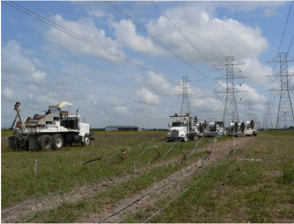
Wire Pulling and Tensioning Site
