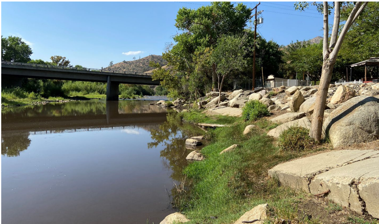
Photograph 6. The Kern River with in-channel vegetation and Bermudagrass turf along the Kern River bank, and broken concrete and imported rock for scour protection, facing south. September 13, 2022.
