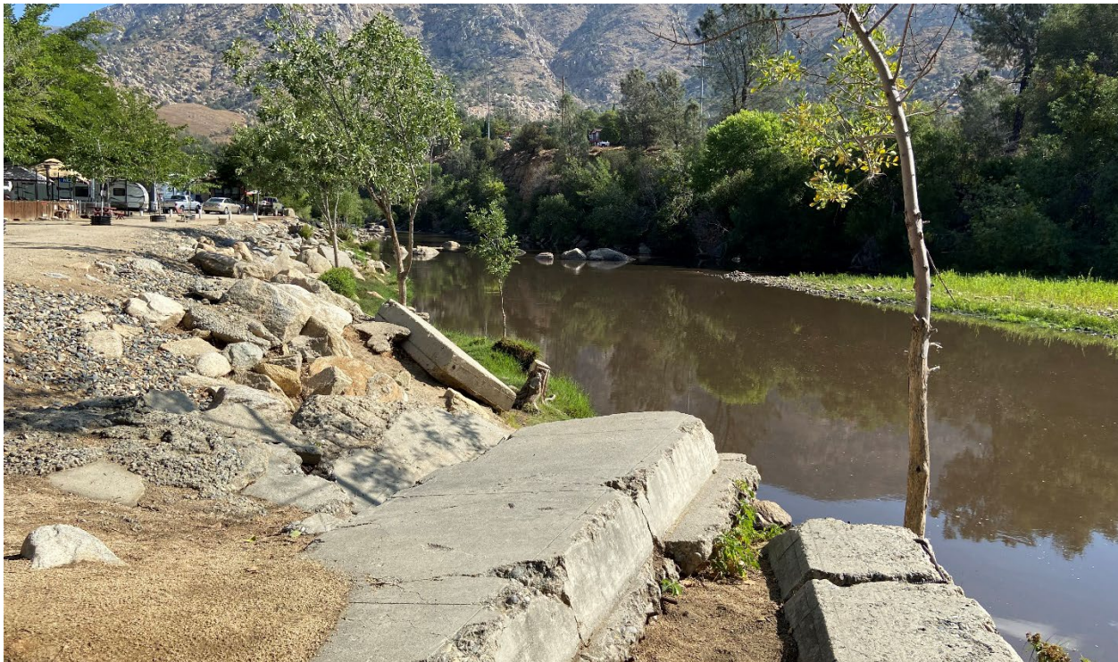
Photograph 4. Broken concrete and imported rocks with landscaped trees for scour protection along the Kern River bank slope, facing northeast. September 13, 2022.
