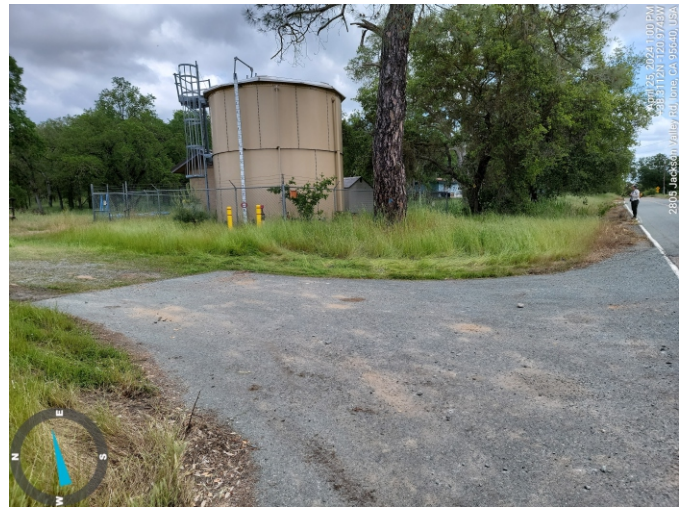
Photo 4: Existing tank off Jackson Valley Road.
