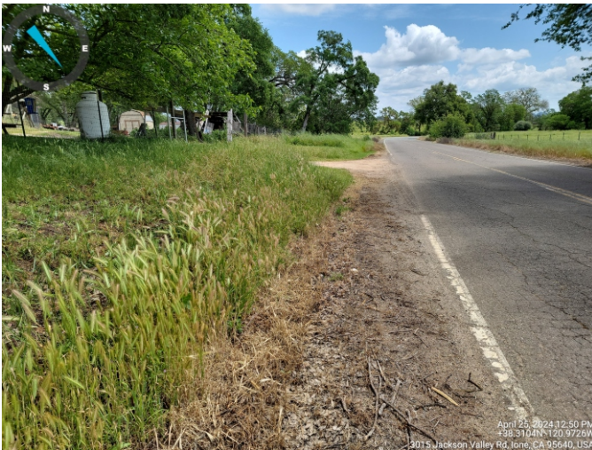
Photo 3: An existing water main is located under Jackson Valley Road.
