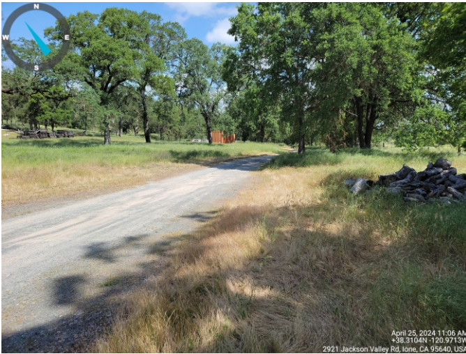
Photo 1: View of typical roadway in which mainline will be installed.
