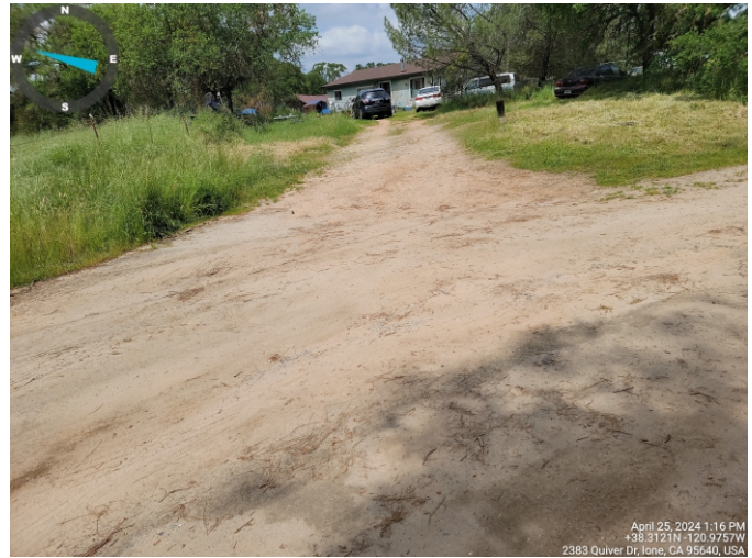
Photo 2: Service lines to individual homes will be installed in driveways.
