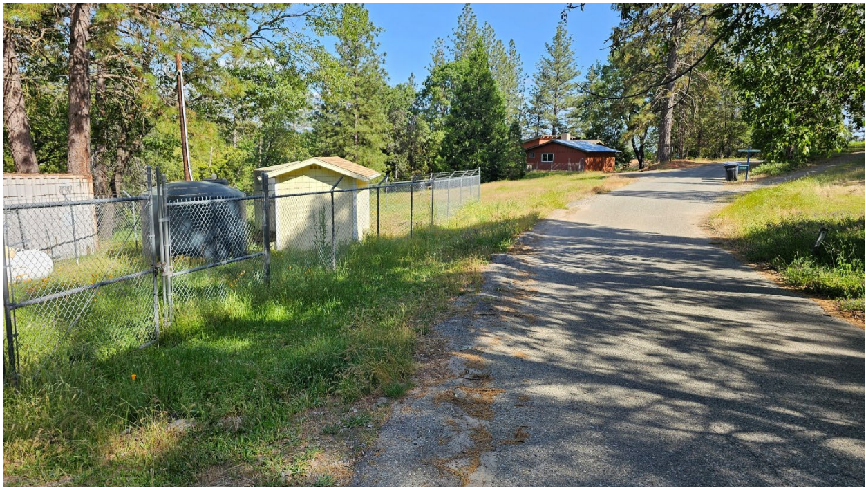
Photo 2: Study area with existing water treatment facilities on left.
