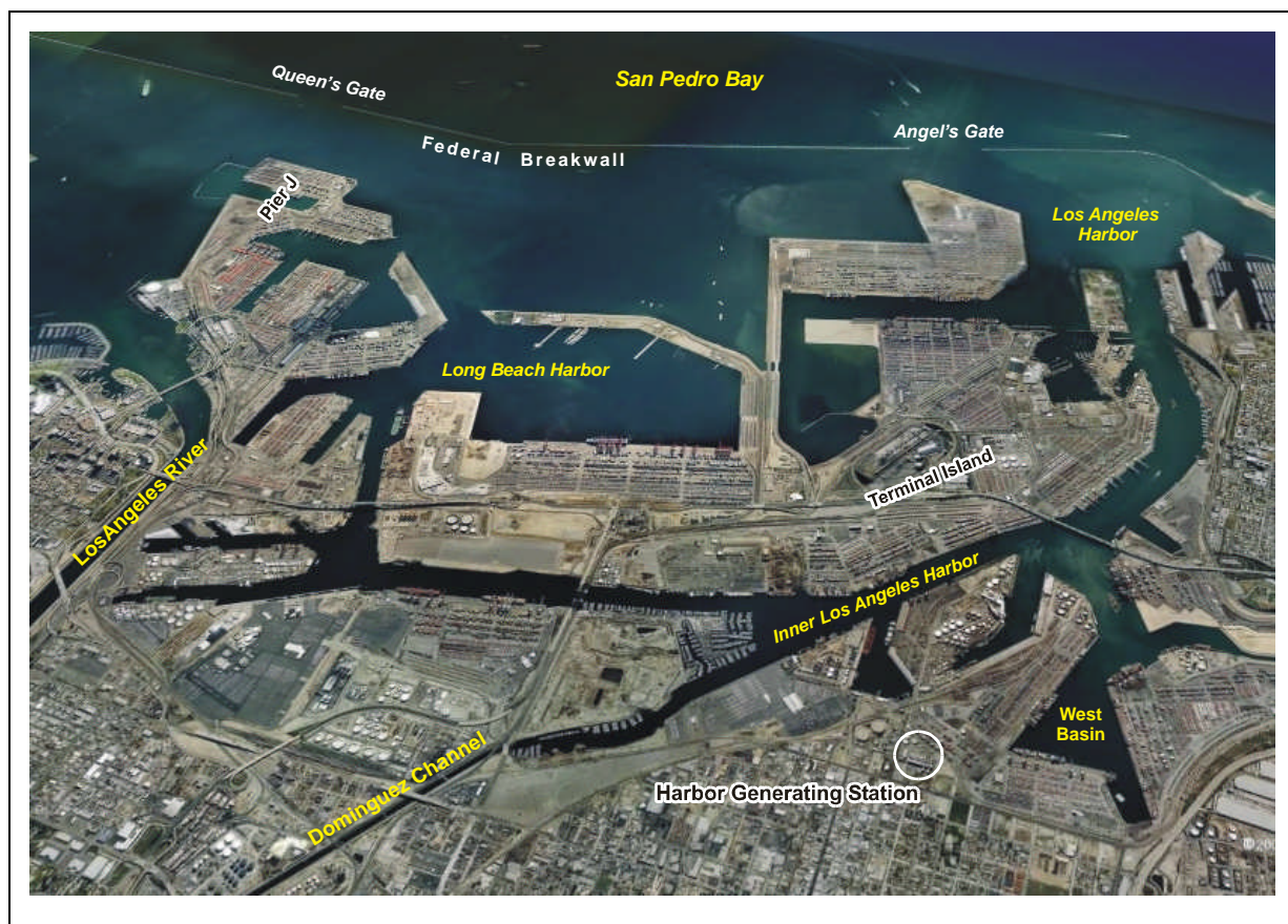
Figure 3.3-1. Aerial view (looking south) of Harbor Generating Station and the vicinity of Los Angeles and Long Beach Harbors.
