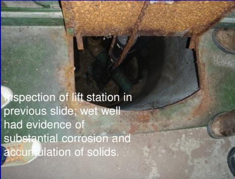
Inspection of lift station in previous slide; wet well had evidence of substantial corrosion and accumulation of solids.
