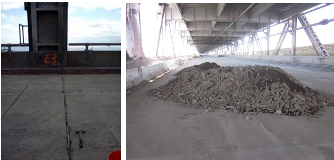
Figure 1-1. PCB-containing Caulk: PCB-containing caulk between road decks of the San Francisco Oakland Bay Bridge Old East span as discovered on inspection (left) and in a pile after removal (right), commingled with asphalt-concrete grindings.
