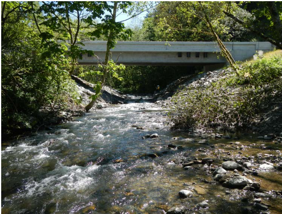
Little Mill Creek (District 1, Eureka), Emergency Bridge Project
