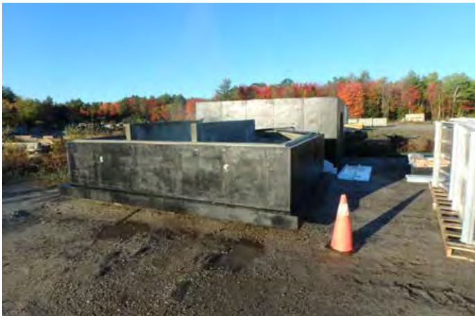
Pre Installation Inspection at Precast Facility
