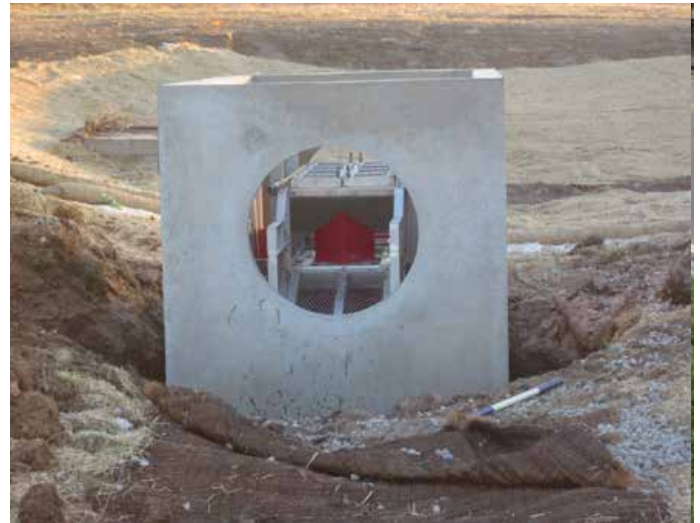
Structure and NSBB™ Internals Set at Install Site
