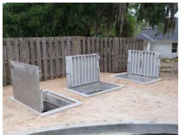
Finished NSBB™ with Hatches Open
