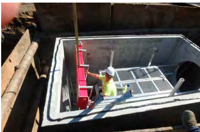
Installation of SkimBoss® Floating Skimmer Panel
