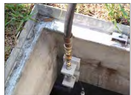
HydroSlide™ quick connector with vacuum truck water supply hose attached for sediment removal.
