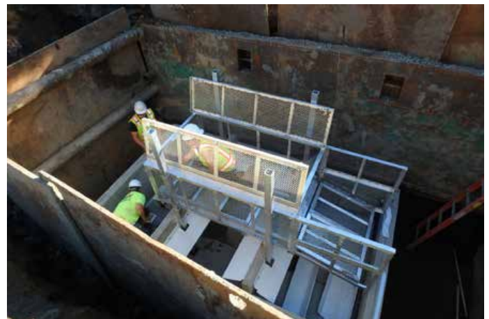
Installation of Screen System
