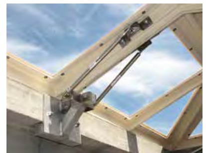
09 Attach center bracket
