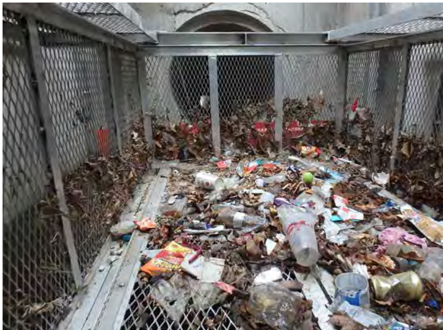
Nutrient Separating Baffle Box ® with collected trash, organics and debris inside the screened basket system ready for disposal.
