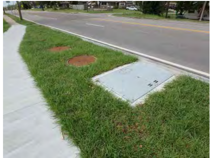
Finished NSBB™ with Manhole / Hatch Configuration
