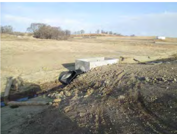
Installation of Pipe Connections
