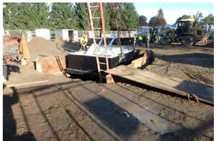
Installation of NSBB™ Base Section
