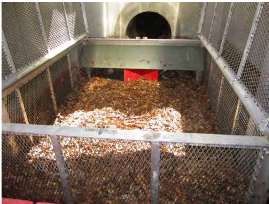
Nutrient Separating Baffle Box® with trash / debris collected inside the screening system basket.
