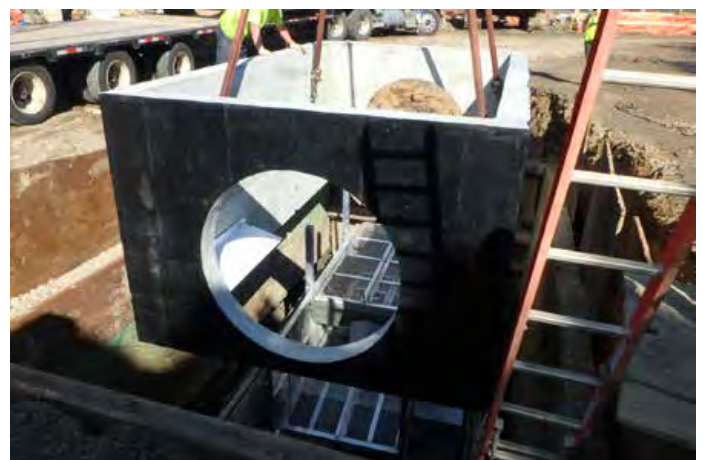
Installation of NSBB™ Treatment Mid Section
