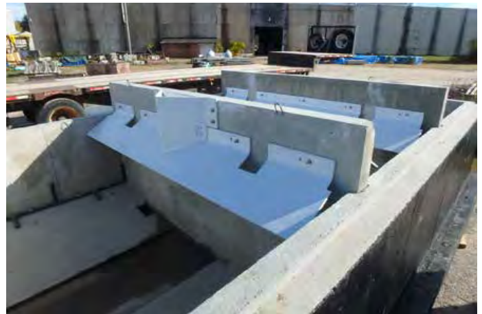
Pre Installation of Turbulence Deflectors
