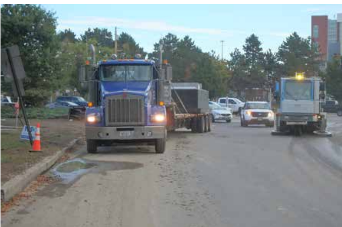
Delivery of Precast Vault to Installation Site
