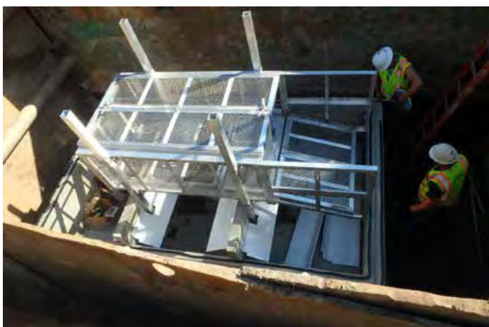
Application of Butyl Tape Sealant Layer to Base Edge
