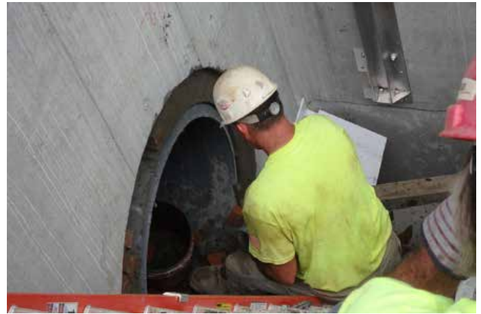
Connection and Grouting of Inflow / Outflow Pipes
