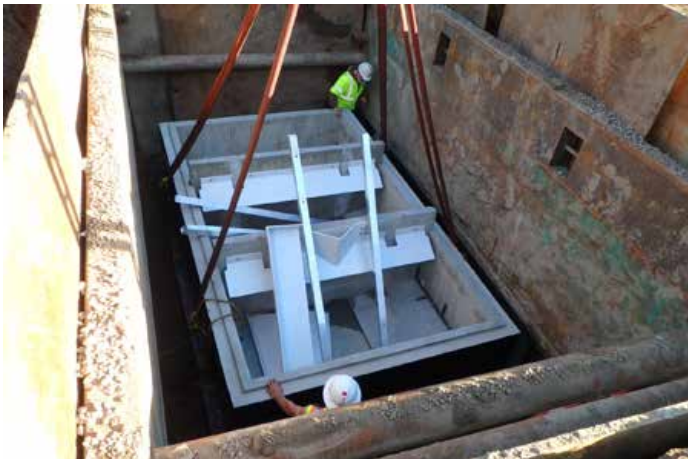
NSBB™ Base Section Installed
