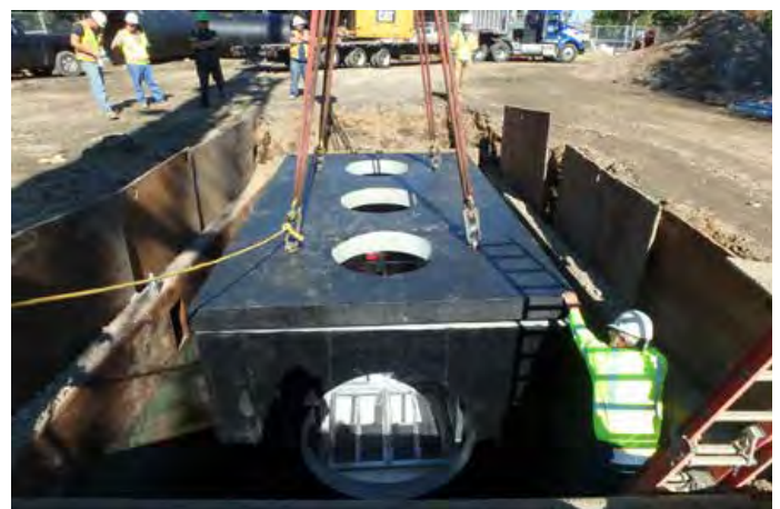
Installation of NSBB™ Top Finishing Slab
