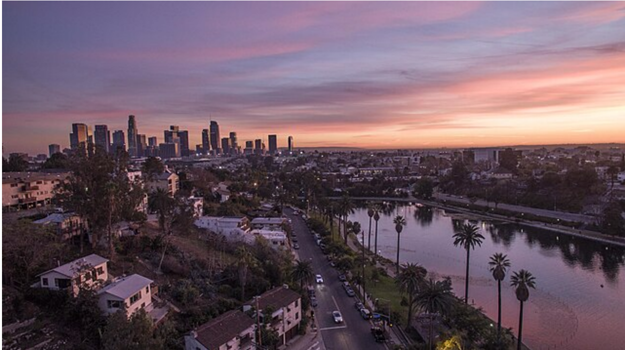
Figure 2: Echo Park Lake in Los Angeles, a multi-benefit stormwater pond.
