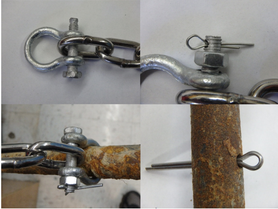
Figure 19. Detail of shackle attachment to stake
