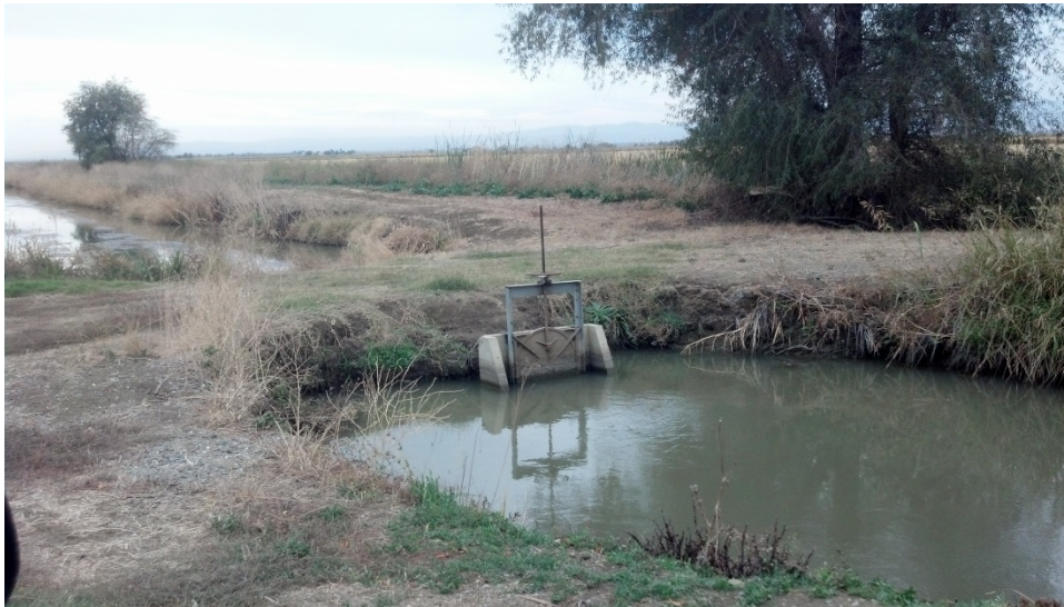
Figure 4.2.32. Water control structures in the Colusa Basin Wildlife Refuge.
