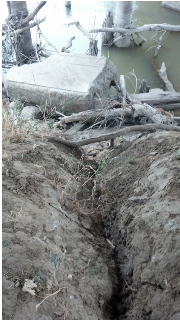
Figure 4.2.20. Evidence of gully erosion on the east bank (river left) of the CBD under the Tule Rd. Bridge.
