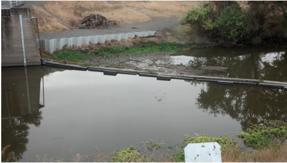
Figure 4.2.5. Stagnant water behind the CBD outfall gates viewed the east levee.
