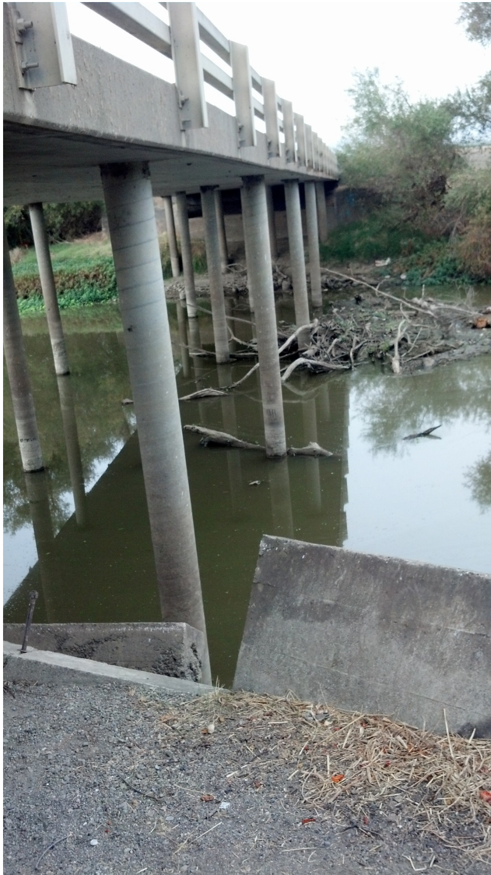
Figure 4.2.13. The County Line Bridge and woody debris as viewed from the concrete abutment at the base of the east levee of the CBD.
