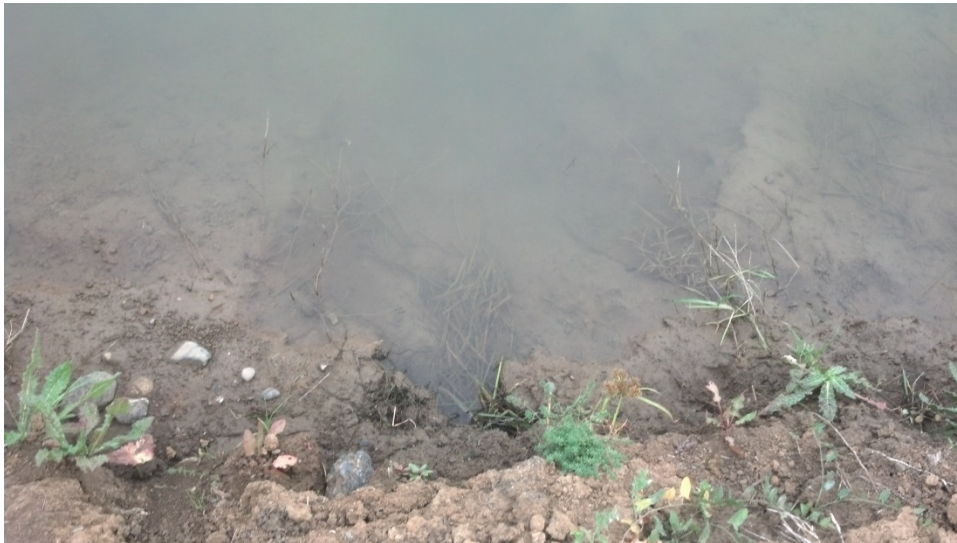
Figure 4.2.50. The earthen channel bank and bottom of the GCID Main Canal.
