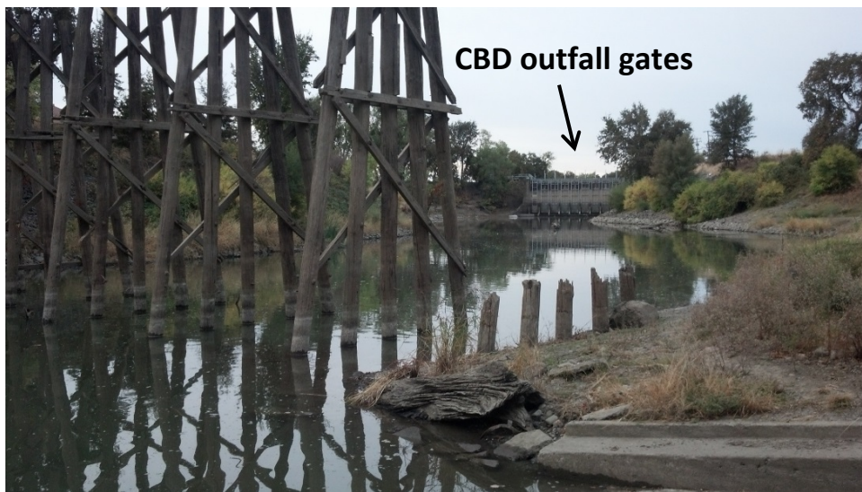
Figure 4.2.4. The CBD outfall gates looking west from the Knights Landing Fishing Access boat launch during Stop 1.
