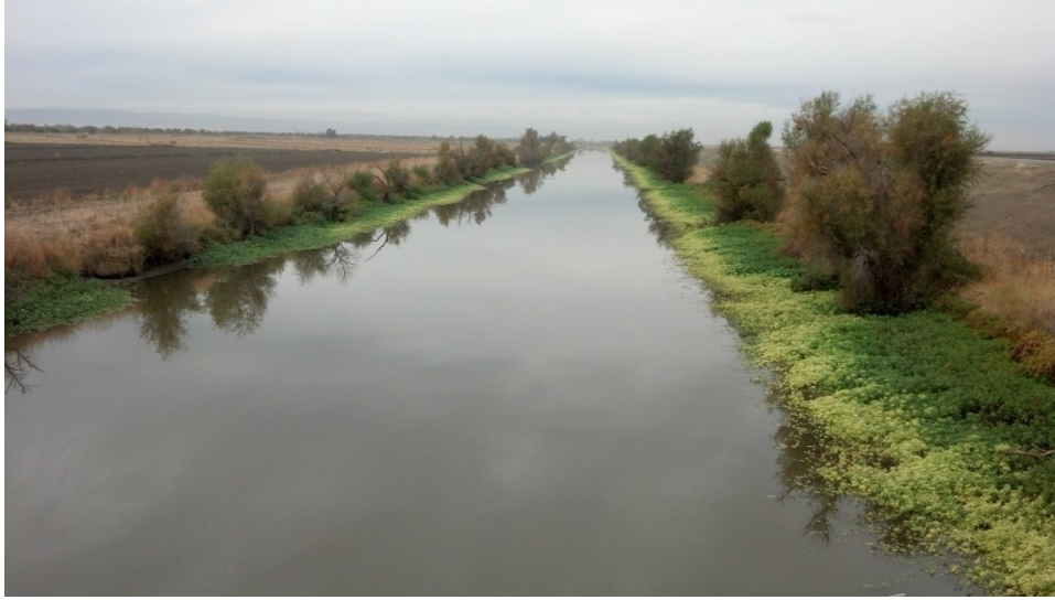
Figure 4.2.9. Still waters of the CBD as viewed in the downstream direction from the Road 99E Bridge.
