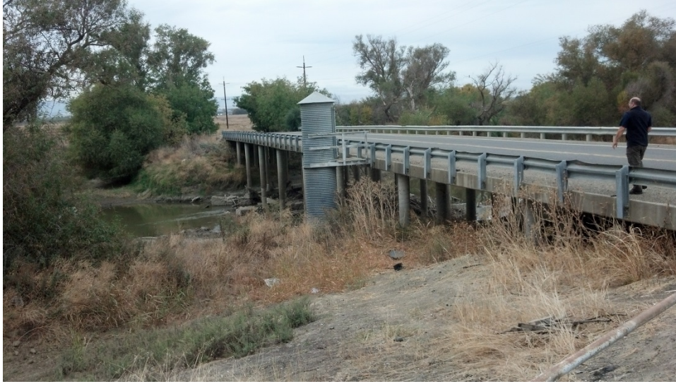
Figure 4.2.17. The Tule Road Bridge over the CBD, which was the location for the UCD/US EPA NPS CBD project's sample site CBD-3 as viewed from the eastern bank (river left) of the CBD. Note apparent stilling well installation for discharge monitoring.
