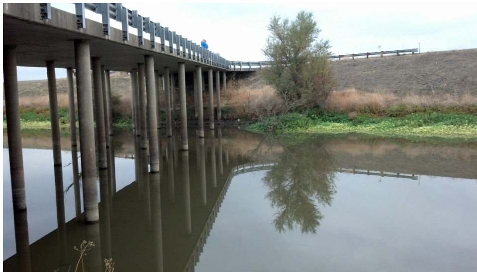
Figure 4.2.8. The Road 99E Bridge as viewed from the base of the west levee of the CBD.
