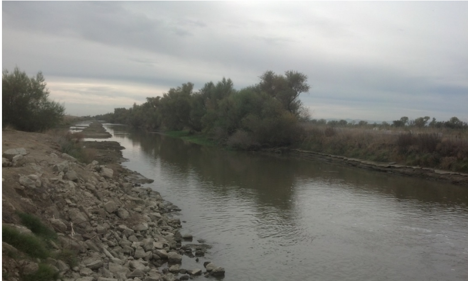
Figure 4.2.29. View of CBD downstream from Davis Weir. Note dual channel reach in upper left quadrant of frame.
