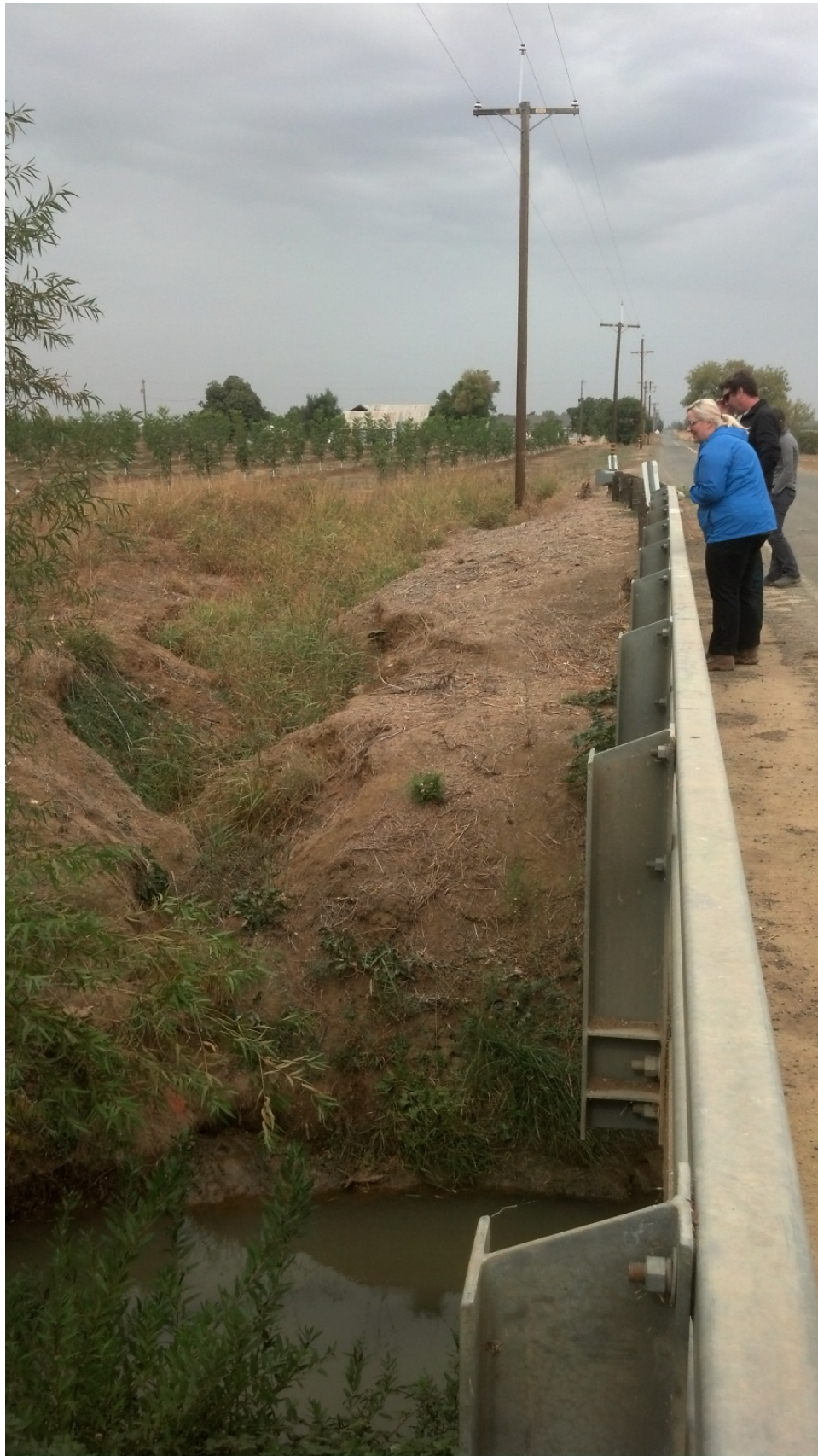
Figure 4.2.36. Stone Corral Creek at the Four Mile Road Bridge. Note large vegetated gully on far bank.
