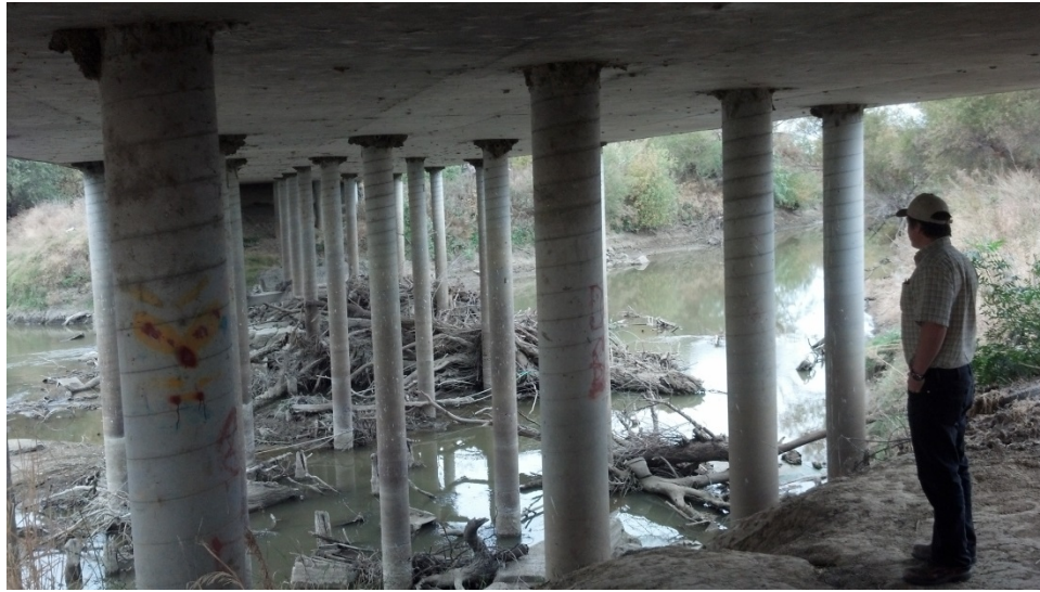
Figure 4.2.19. View of underside of Tule Rd. Bridge from east bank (river left) illustrating woody debris jam.
