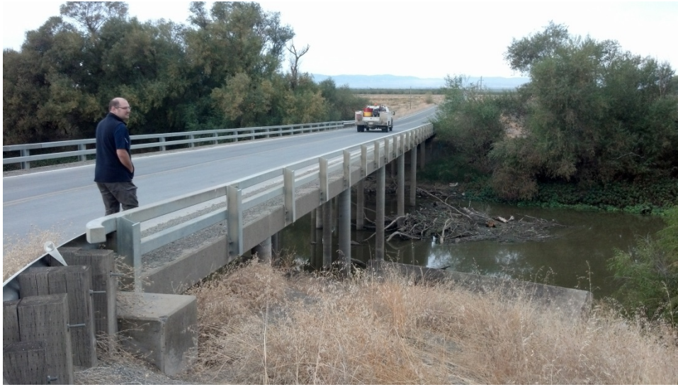
Figure 4.2.12. The County Line Road Bridge over the CBD, which was the location of the UCD/US EPA NPS CBD sampling station CBD-2 as viewed from Road 108 on the east levee of the CBD. Note the deposit of woody debris and sediment against the bridge supports in mid-channel.
