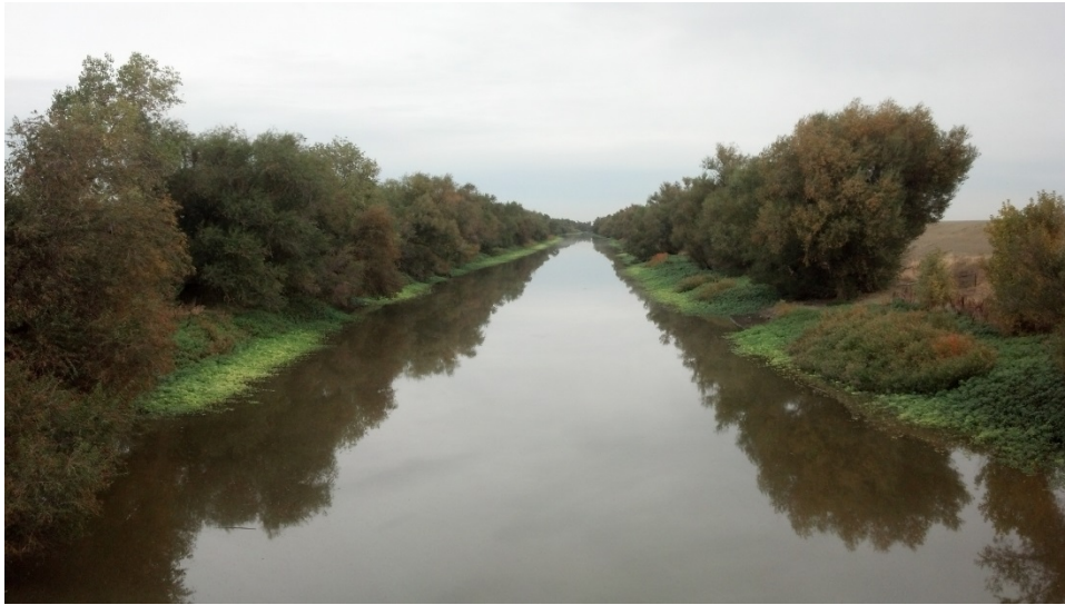
Figure 4.2.14. The CBD channel exhibiting still water conditions as viewed from the County Road Bridge in the downstream direction.
