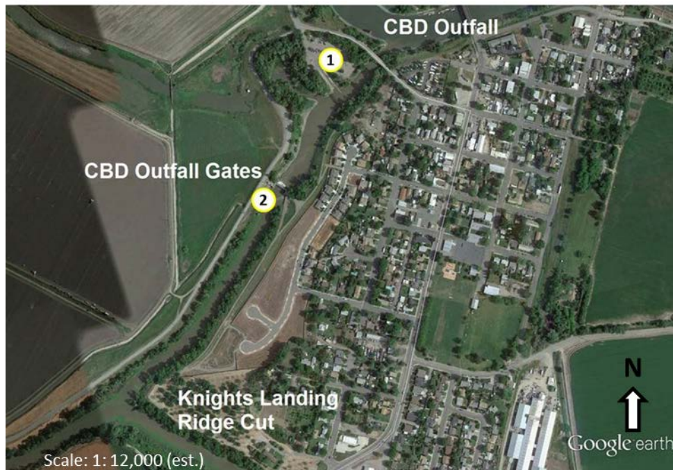
Figure 4.2.1. Stop 1: The CBD outfall into the Sacramento River near Knights Landing. Stop 2: The CBD outfall gates.
