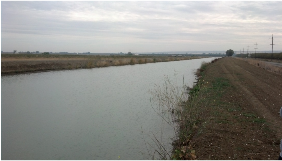
Figure 4.2.49. The GCID Main Canal as viewed from its east bank. Note its earthen construction.
