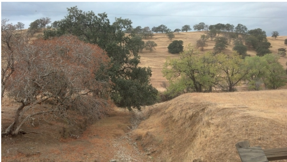
Figure 4.2.46. The dry bed of Antelope Creek as viewed from river right with incised thalweg, and steep right bank with grass cover and bare earth.
