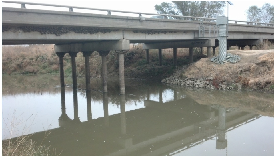
Figure 4.2.34. The Highway 20 Bridge over the CBD, which was the location of the CBD-5 sampling site during the UCD/US EPA NPS CBD project, and continues to be the location of the DWR hydrologic gauging station A02876, as viewed from river right. Samples have also been collected here under CVRWQCB programs (station 520COL006). Note the presence of surface currents visible downstream from the central bridge supports.
