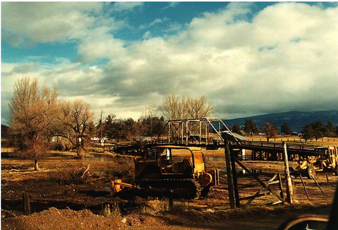
Figure 4. This photograph shows heavy equipment and excavation in the riparian zone of the Shasta River above Louie Road just upstream of the convergence with Big Springs Creek in January 1995. From Klamath Resource Information System V 3.0 (TCRCD, 2003).
