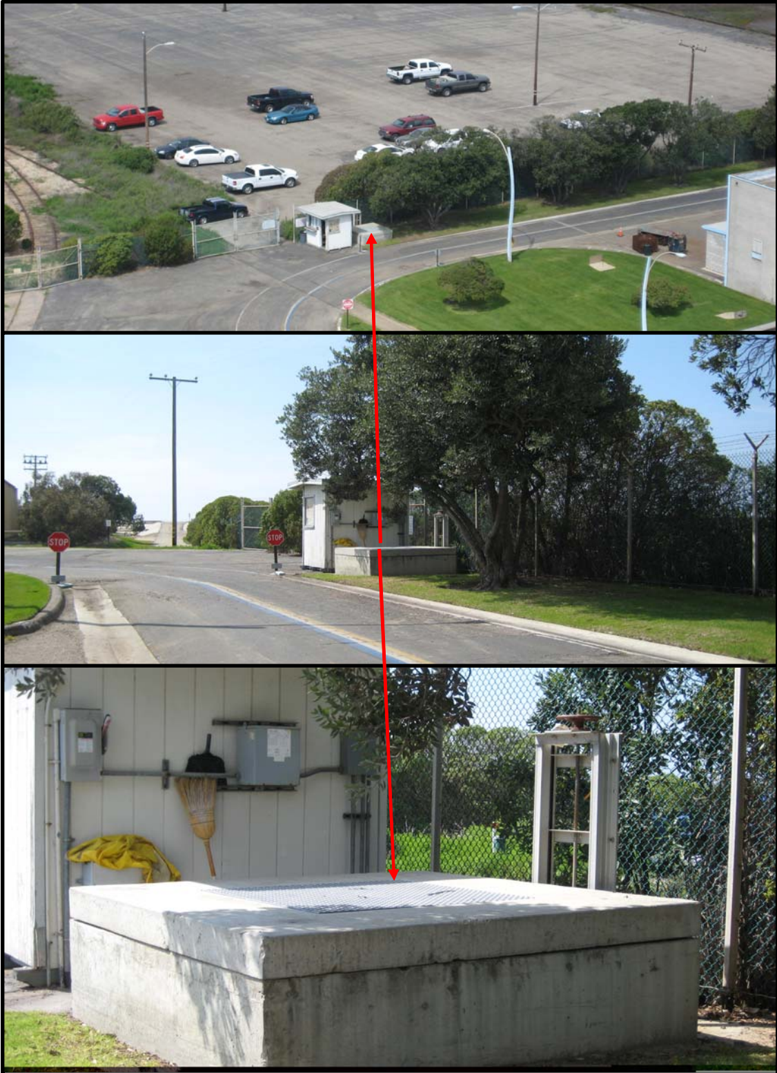
Figure 2.5.7. Stormwater collection points D5 - D12 North East Yard Drain east of contractor's gate.
