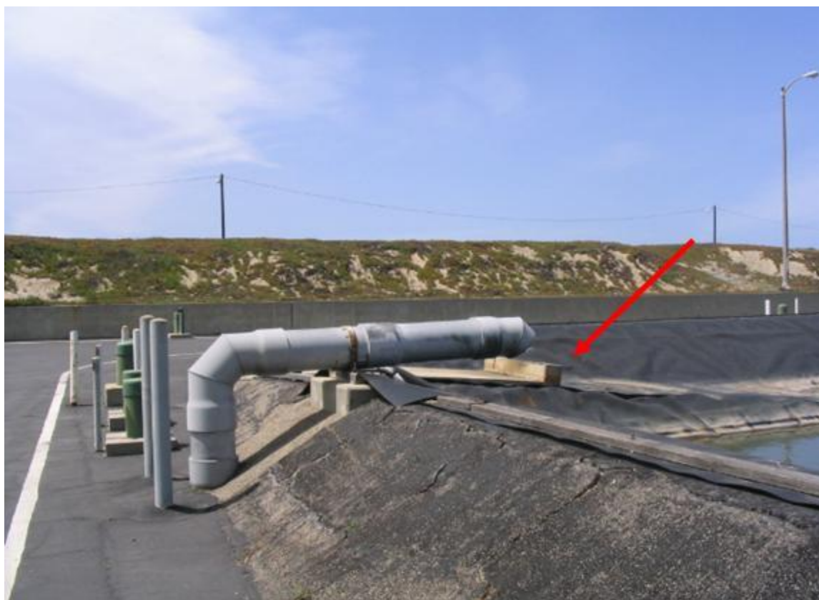
Figure 2.5.8. NPDES Storm Water Retention Basin South.
