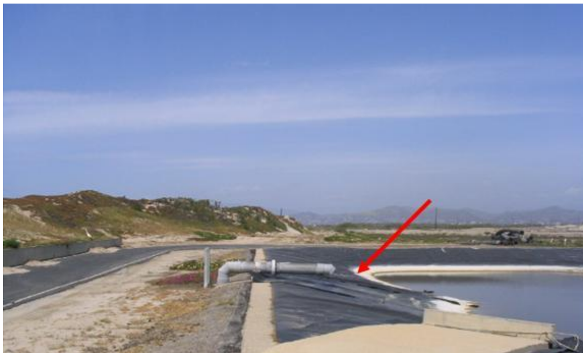
Figure 2.5.7. NPDES Storm Water Retention Basin North.
