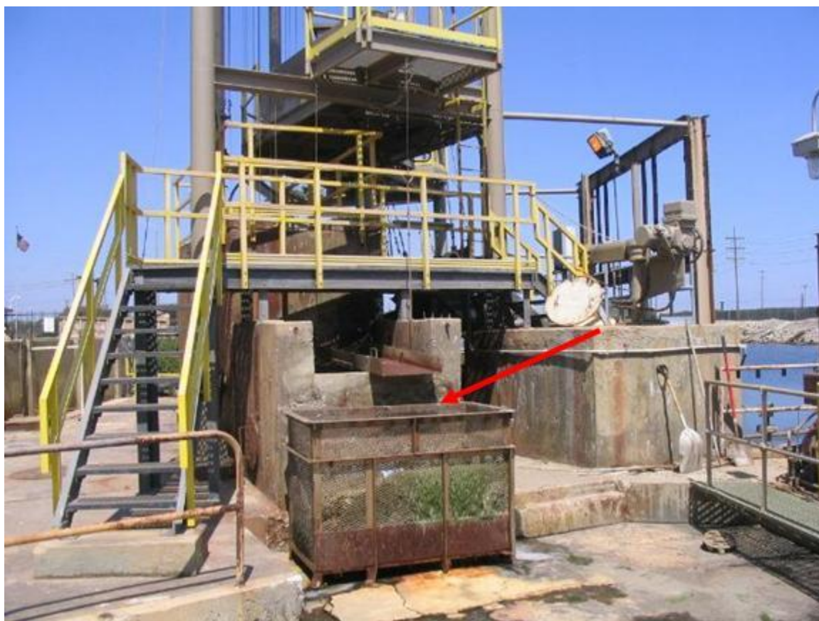
Figure 2.5.9. NPDES fish impingement collection point.
