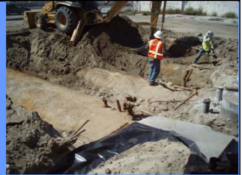
Photo 3: USTs being excavated.
