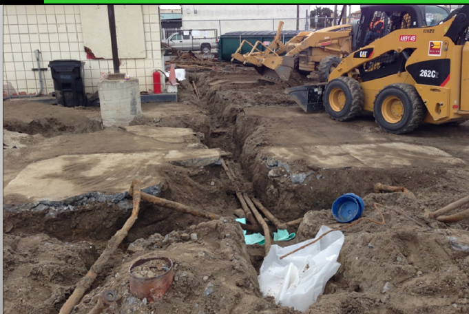
Photo: Removal of product piping at a former gas station
