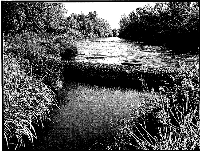
View upstream on the Merced River showing the Point of Rediversion at the Ruddle Ditch Diversion Structure
