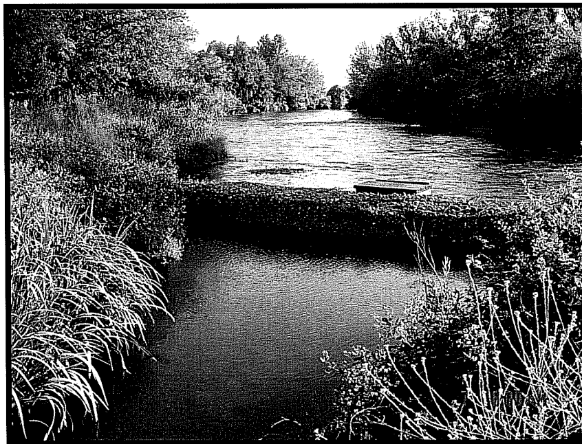
View upstream on the Merced River showing the Point of Rediversion at the Ruddle Ditch Diversion Structure
