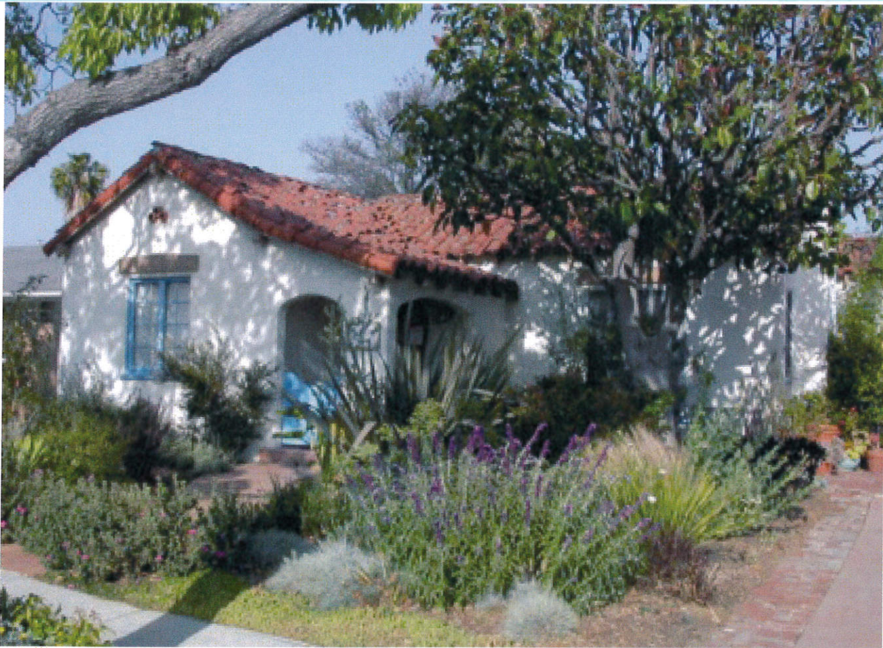
Drought-tolerant yard in the EBMUD service district
