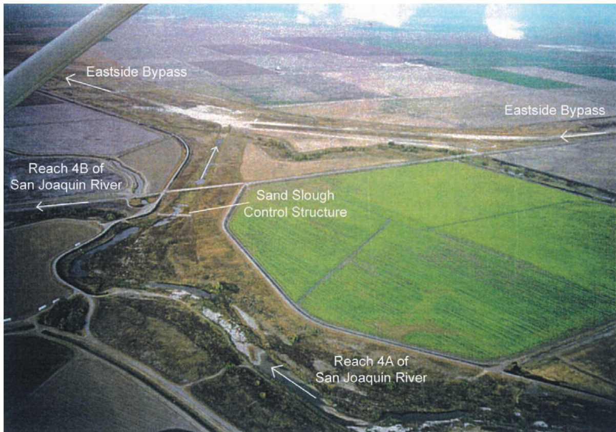
Figure 3-50. View looking downstream at the Sand Slough control structure reach of the San Joaquin River at RM 168. The San Joaquin River upstream of the structures bifurcates into San Joaquin River (left channel, well vegetated banks), Sand Slough (center channel, unvegetated banks), and the Eastside Bypass. Note sediment deposit deposition in the bypass channel. Design capacity of the bypass channel is about 16,500 cfs. From JSA and MEI (1998).
