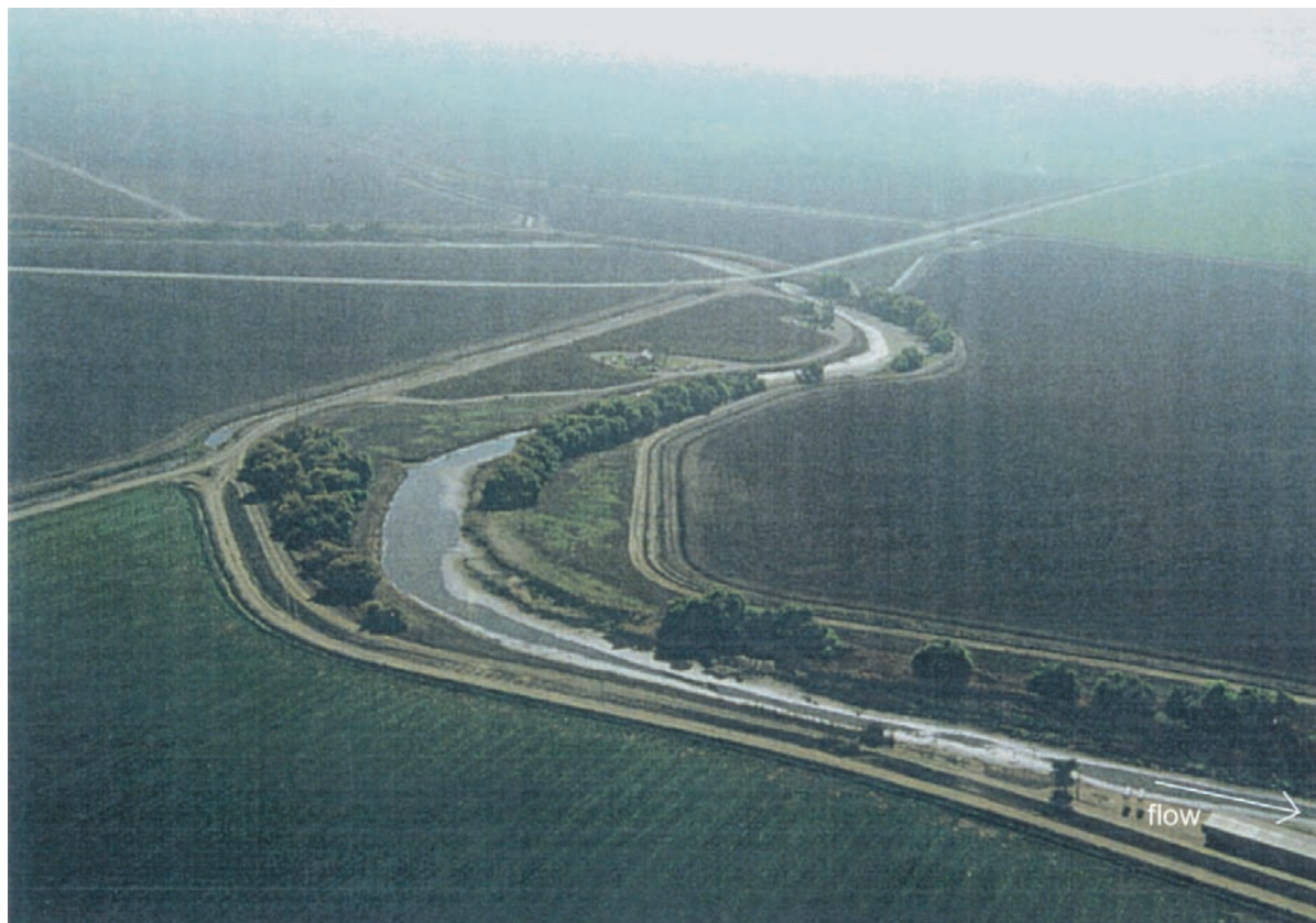
Figure 3-51. View looking upstream at the San Joaquin River at Turner Island Road crossing, RM 157. Design capacity of the channel and levees is about 1,500 cfs; however, actual capacity in many portions of this reach is much less. From JSA and MEI (1998).
