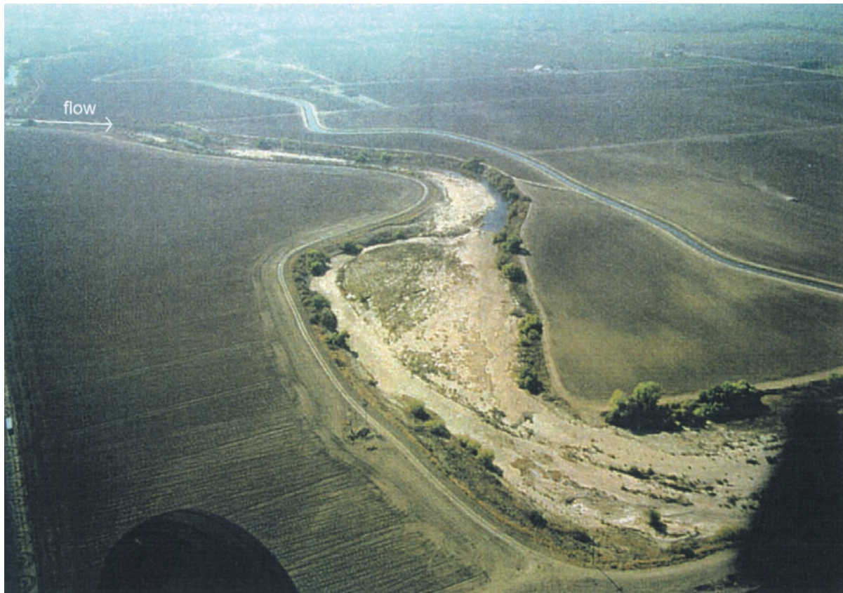
Figure 3-49. View looking upstream at sediment deposition in the bed of the San Joaquin River at about RM 175. Much of the sand appears to be derived from bank erosion. The within-levee capacity in this reach of the river is about 4,500 cfs. From JSA and MEI (1998).
