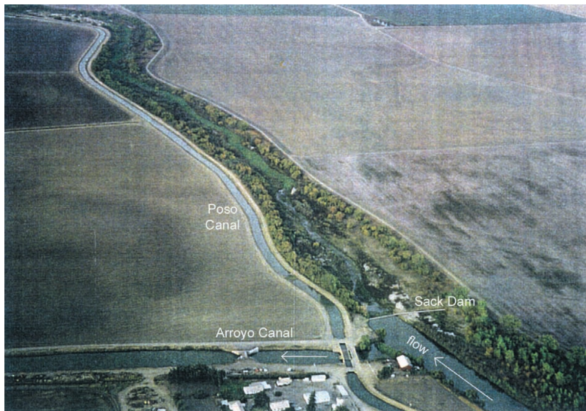
Figure 3-41. View looking downstream of Sack Dam and the headgates for the Arroyo Canal at RM 182. The dam is the terminus for Delta-Mendota water conveyed down the San Joaquin River. The Poso Canal parallels the river on the left bank. From JSA and MEI (1998).
