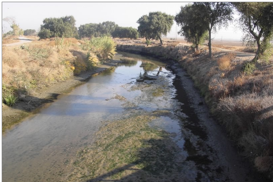
Figure 12 Middle River at Undine Bridge Photo 1
