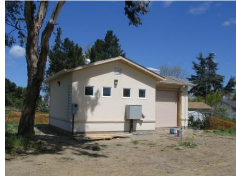
Additional well fields, like the one housed in this building in Campbell, may be one approach to improving infrastructure reliability.
