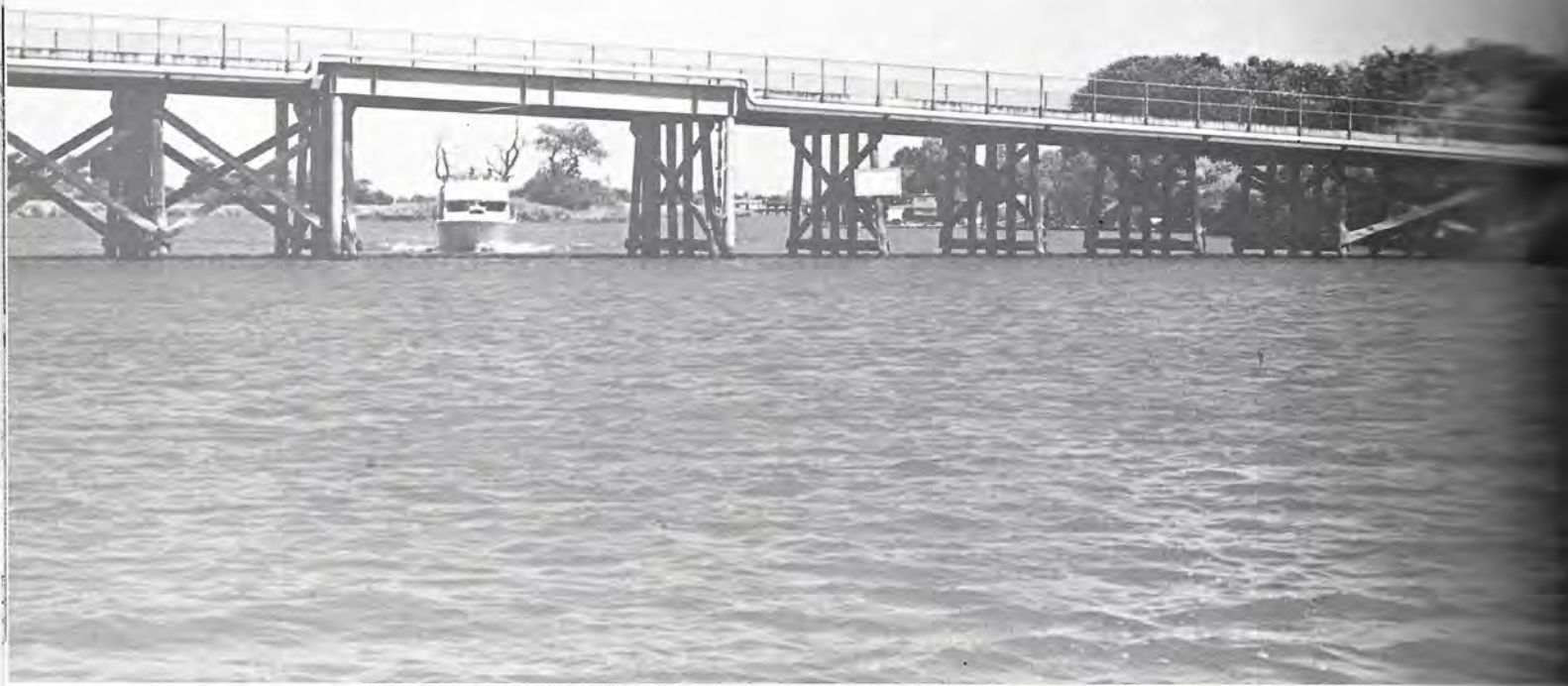
The Jersey Island bridge over Dutch Slough.
