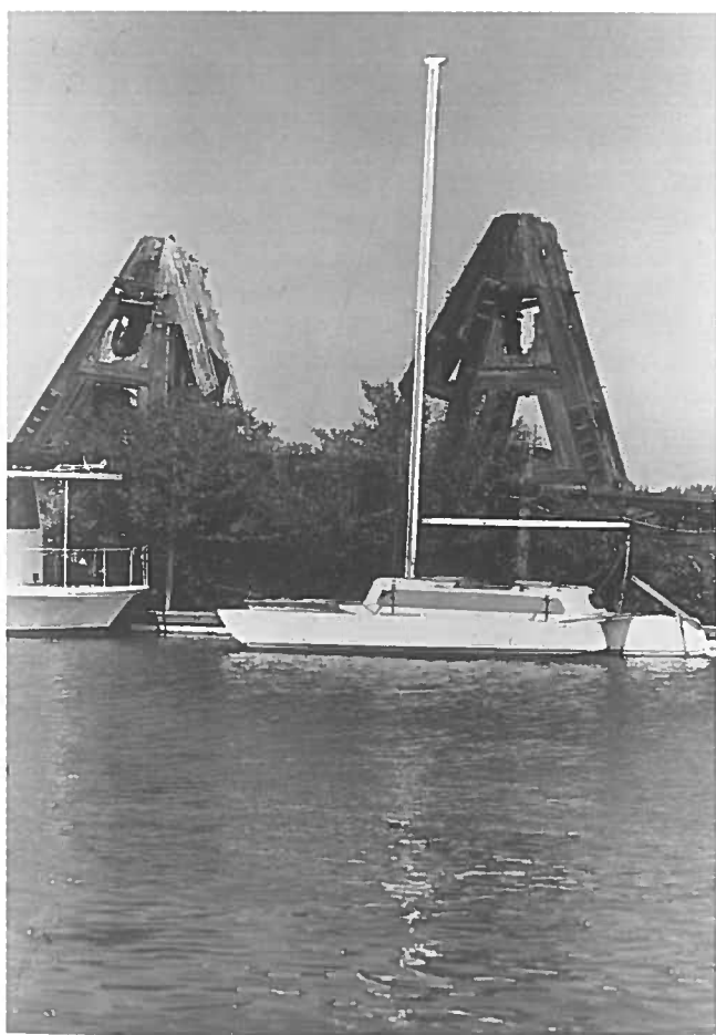
Rodgers Point Marina with the remains of the Solano in the background.
