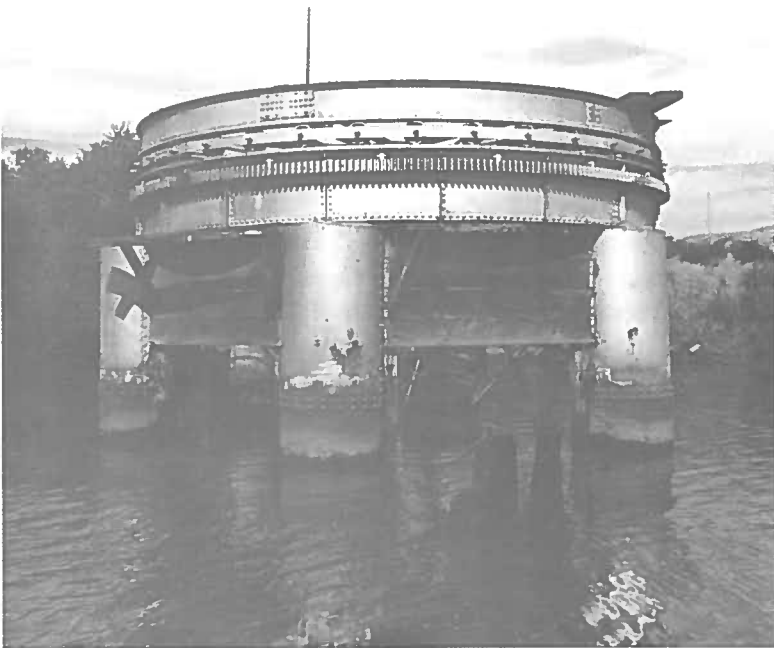
Remains of an old drawbridge on Burns Cutoff.
