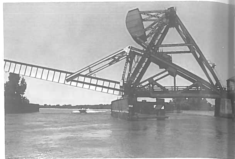
An Old River bascule-type railroad bridge.
