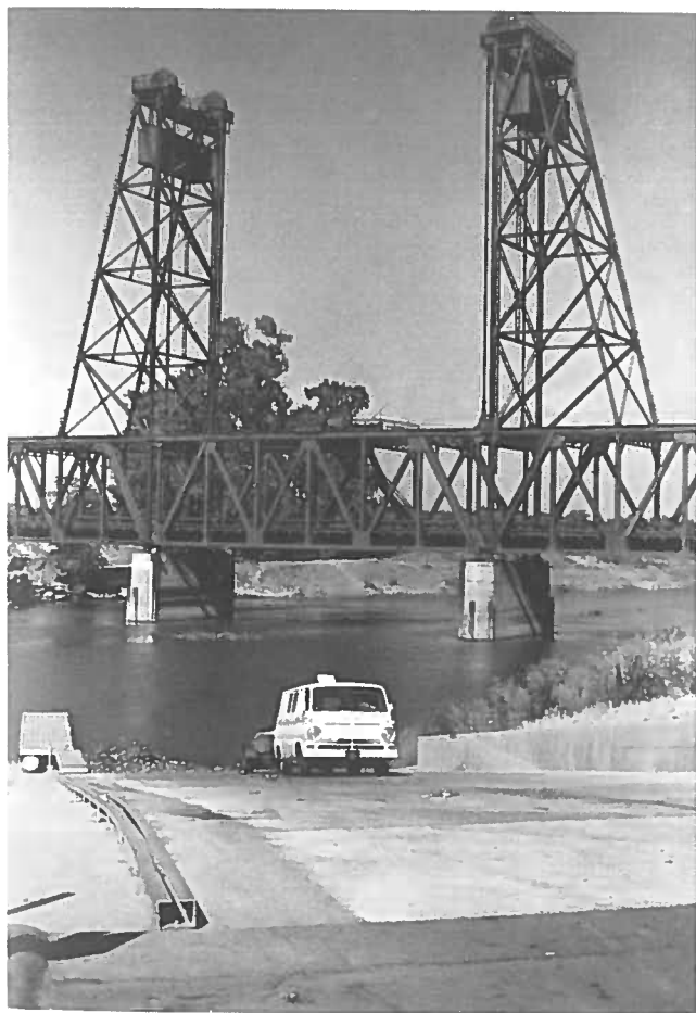
Launching at Mossdale Crossing.
