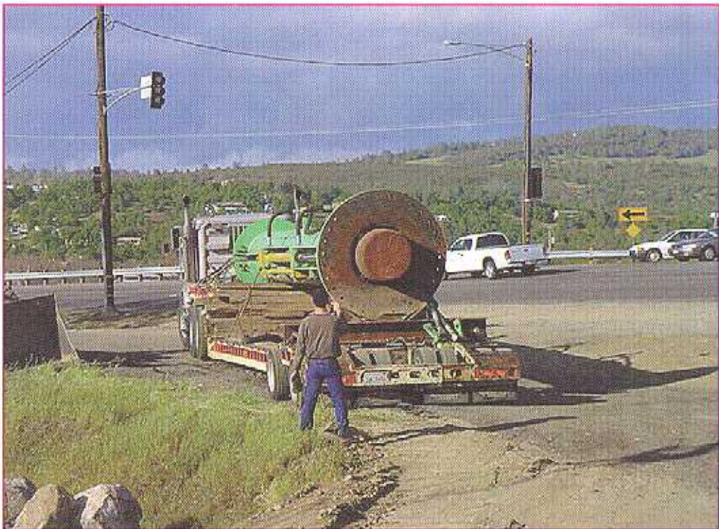
The LMC 50 hydraulic impact hammer, designed and built by Lucas Marine, is delivered to the Putah Creek job site.
