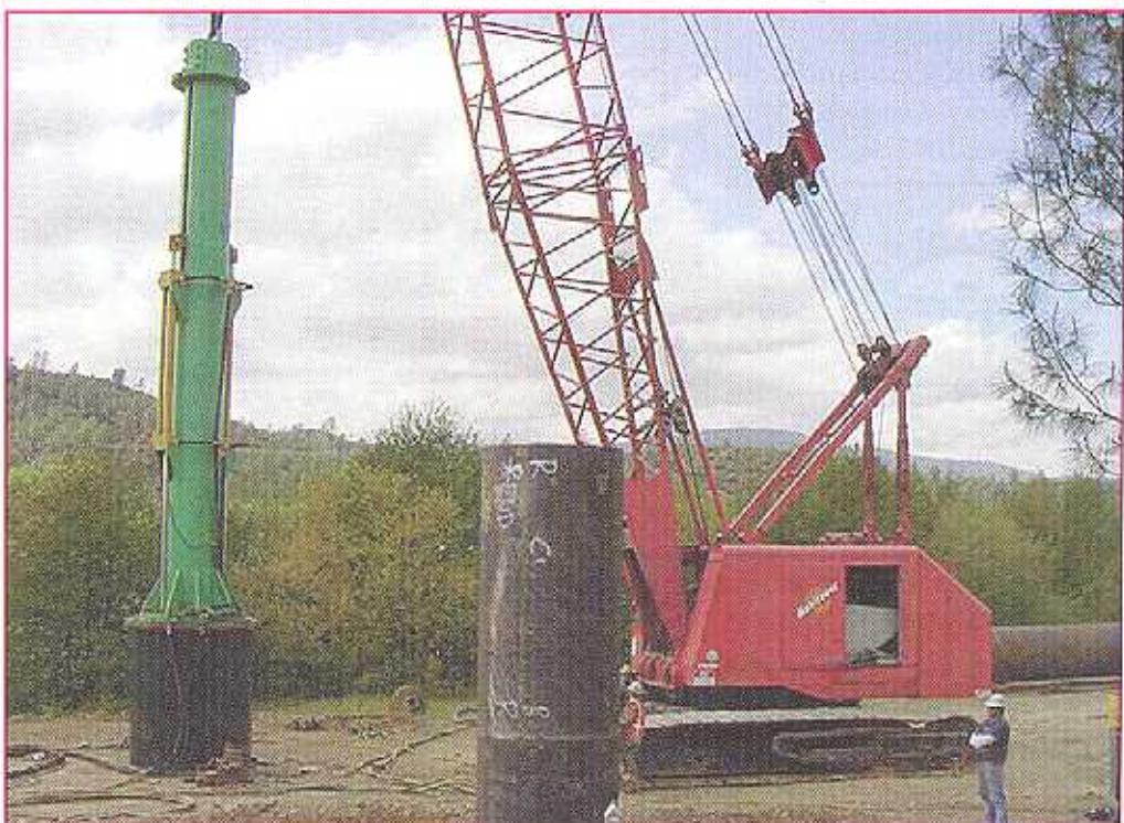
Lucas Marine's LMC 50 hydraulic impact hammer driving a 60-inch pile for the Putah Creek bridge.
