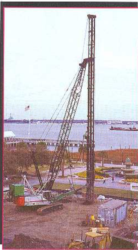
A Link-Belt LS-138 H II doing its job in Charleston, S.C.
