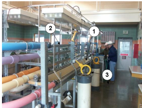
Figure 2-26 PIT Tag Detection and Automated Side Gate
