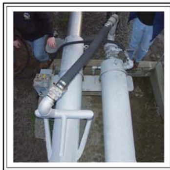
FLUSHING FLOW IS ADDED TO RELEASE PIPE - TYPICAL OF SWP AND CVP RELEASE SITES
