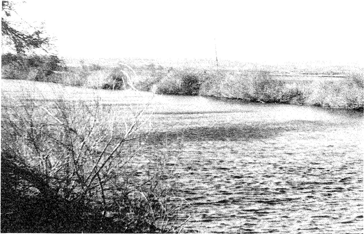
Figure 5. Privately owned and maintained levees on Sevenmile Slough. Note steepness of edge, erosion, and narrow riparian band extending into water.
