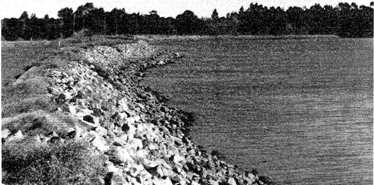
Figure 4. Project levee on north fork of Mokelumne River. Note absence of riparian or emergent vegetation.
