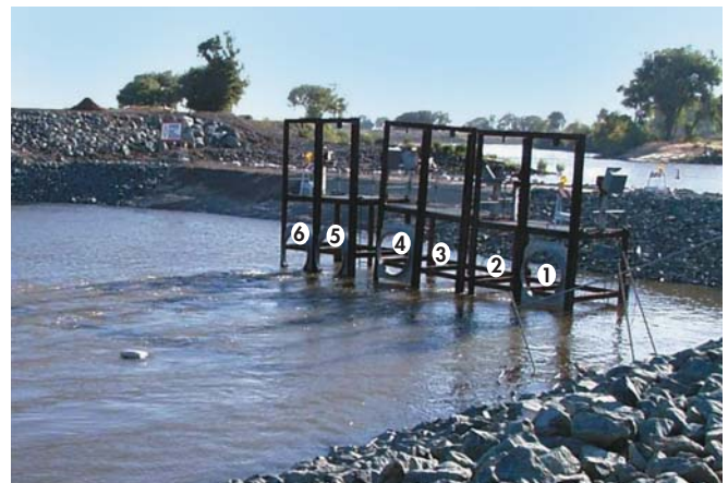
FIGURE 4-2 Culvert Numbers for HORB 2002
