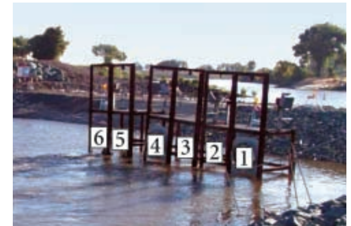
FIGURE 4-2 Culvert Numbers for HORB 2001
