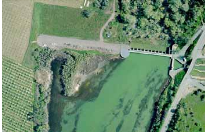
Putah Creek Diversion Dam
