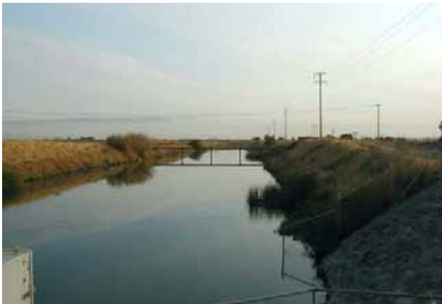
Looking east from Contra Costa Canal Pumping Plant No. 1 at the unlined portion of the canal in the section where local groundwater seepage occurs, which is particularly noticeable at low diversion rates.
