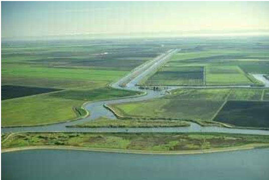
Looking east at Victoria Canal from above Clifton Court Forebay. Victoria Canal is a potential location for CCWD's proposed alternative drinking water intake.
