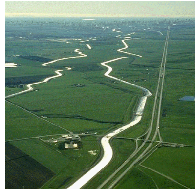
California Aqueduct and Delta Mendota Canal
