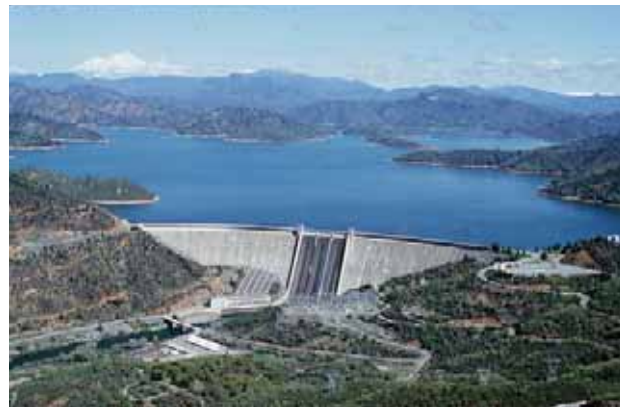
The 4.5 million acre-foot Shasta Reservoir on the Sacramento River near Redding is part of the federal Central Valley Project. Releases from this reservoir play a major role in controlling water quality in the Delta. Raising Shasta Dam and increasing storage in the reservoir are part of the CALFED Surface Storage Program.
