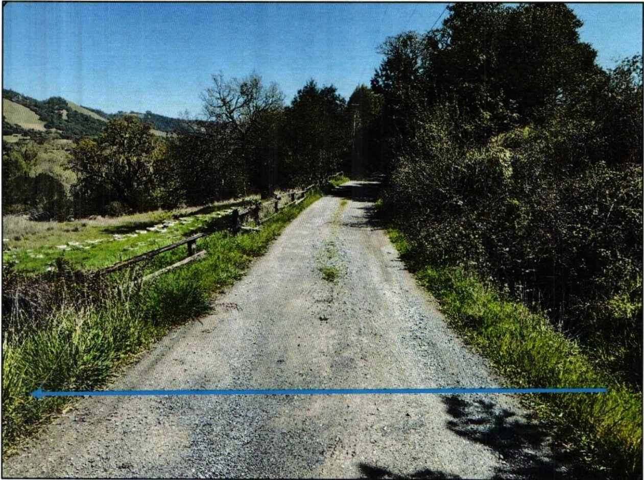
Photo #3 site ID SC-1: Location of the stream crossing beneath the access road. A misaligned culvert conveys flows into the field, visible at the left side of the photo. The approximate culvert location is represented by the blue arrow.
