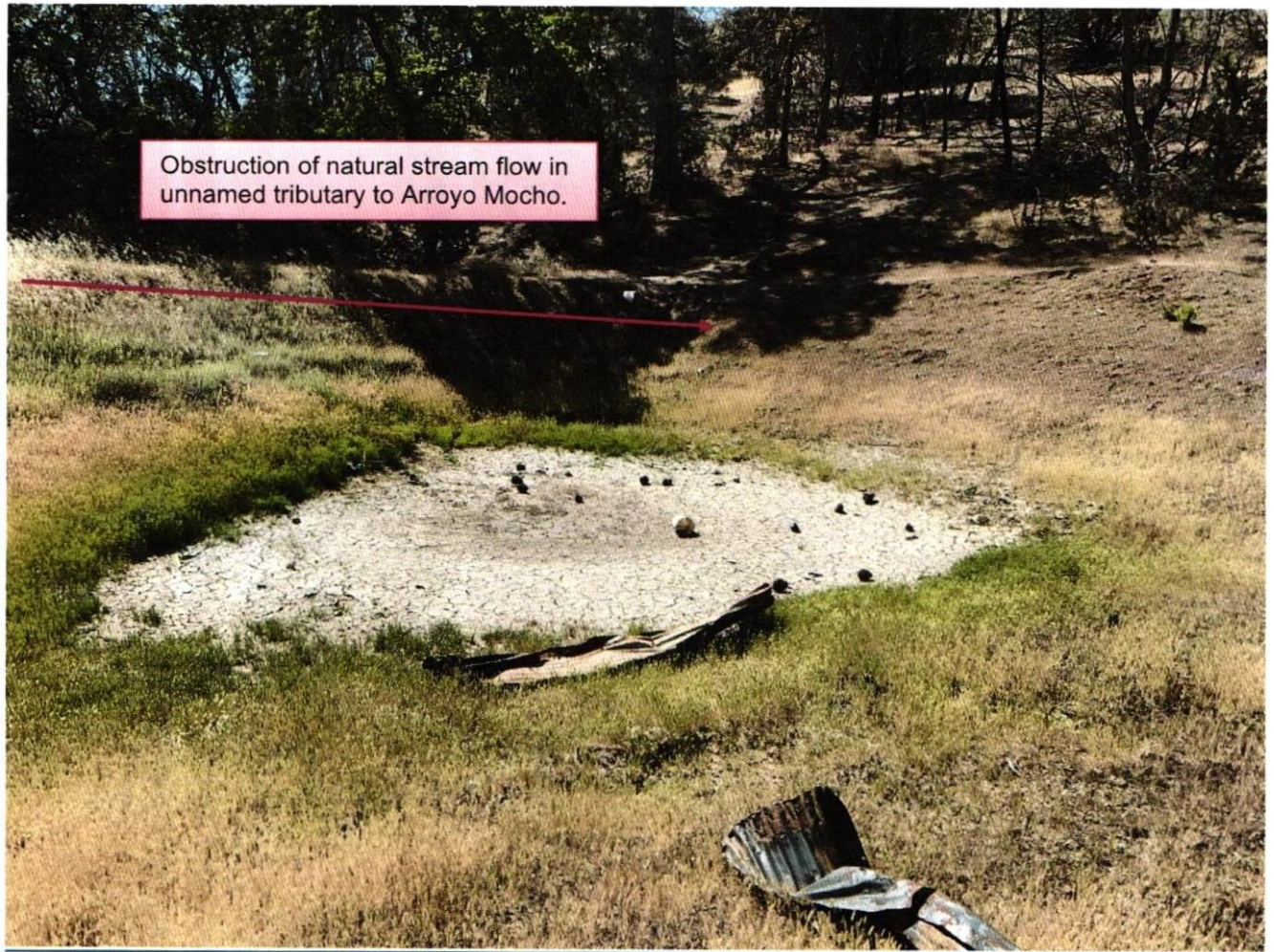
Photo #1, Site ID "HAPt-1". Construction of a dam, placement of fill, and obstruction of natural stream flow in an unnamed tributary to Arroyo Mocho. Creation of onstream reservoir due to obstruction of natural stream flow.
