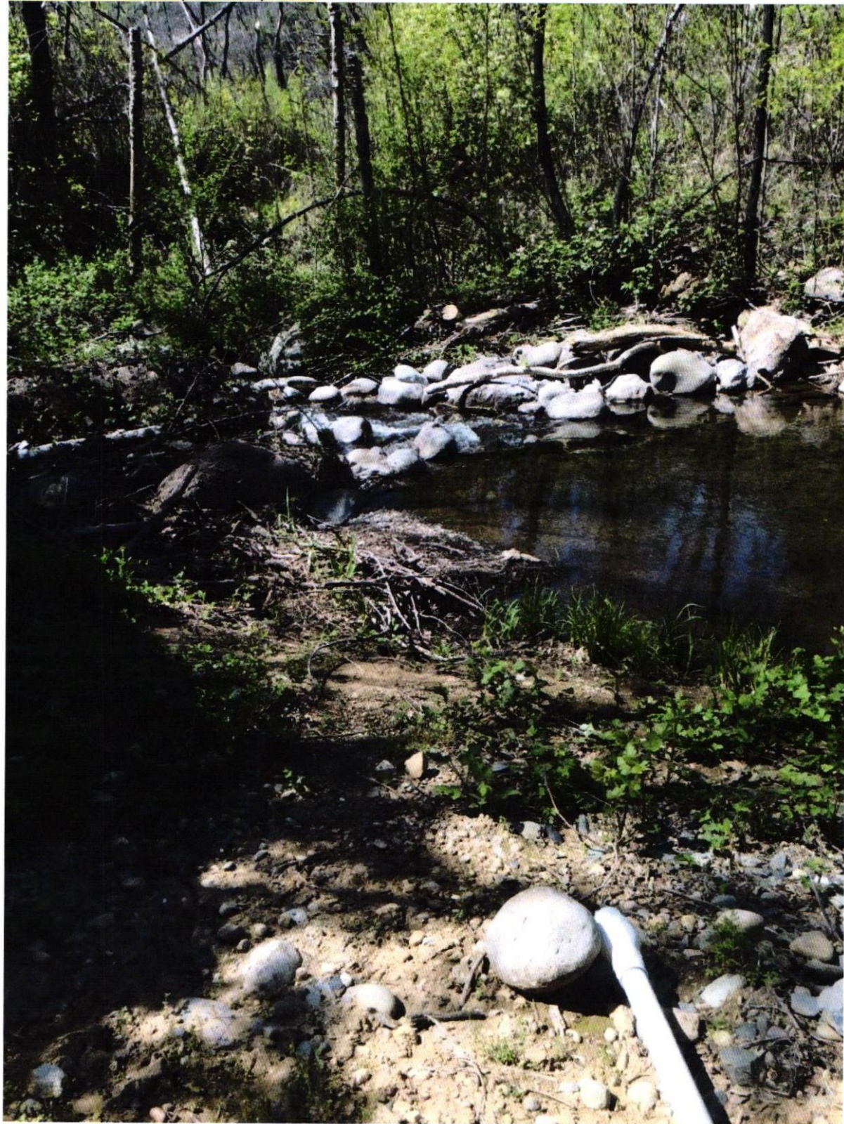
Figure 7: Alteration of the stream bank for access to install a water diversion pipe and pump. Active diversion infrastructure removed prior to inspection.
