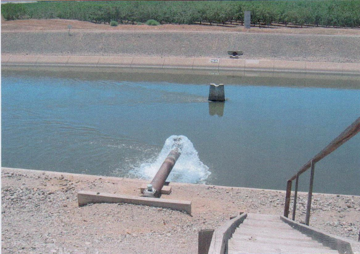
Groundwater Pumped into the DMC near Los Banos, California
