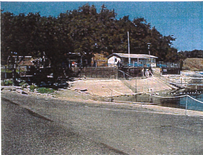
Launch Ramp looking North at Shops
