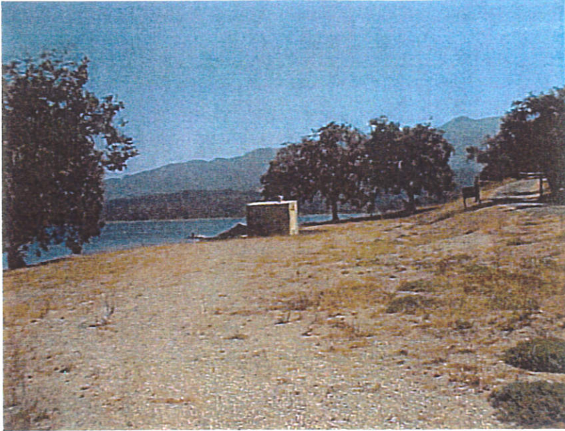
Water Intake Facility looking South
