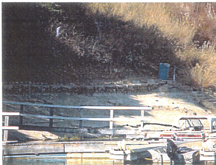
Concrete Lining Erosion control at Access
