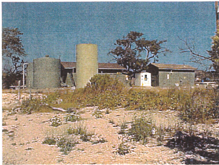
Water Treatment Plant looking East
