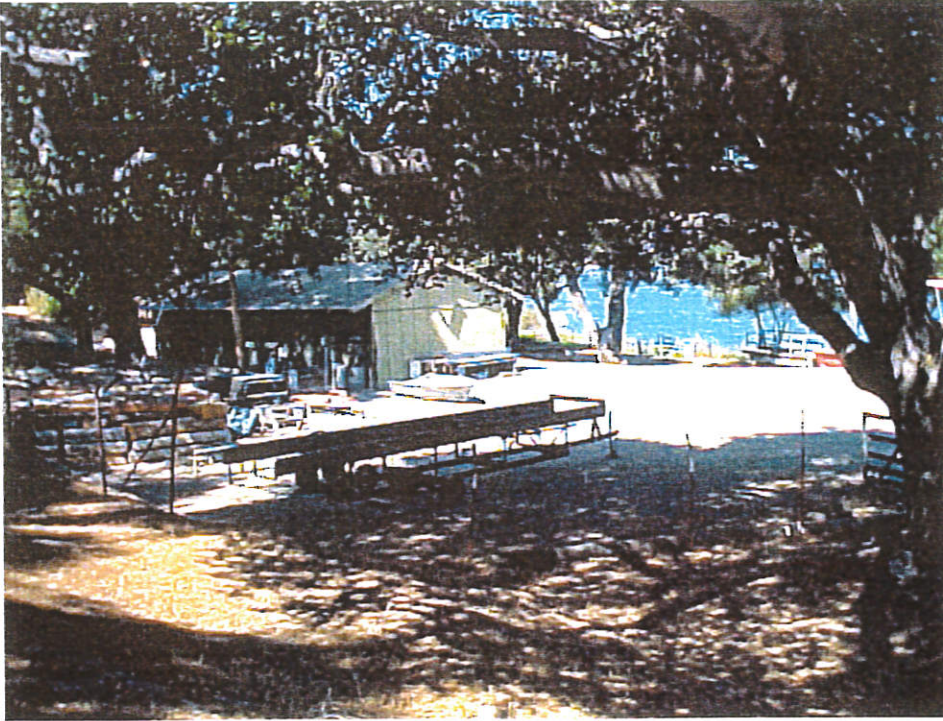
Boat Works Shop looking North
