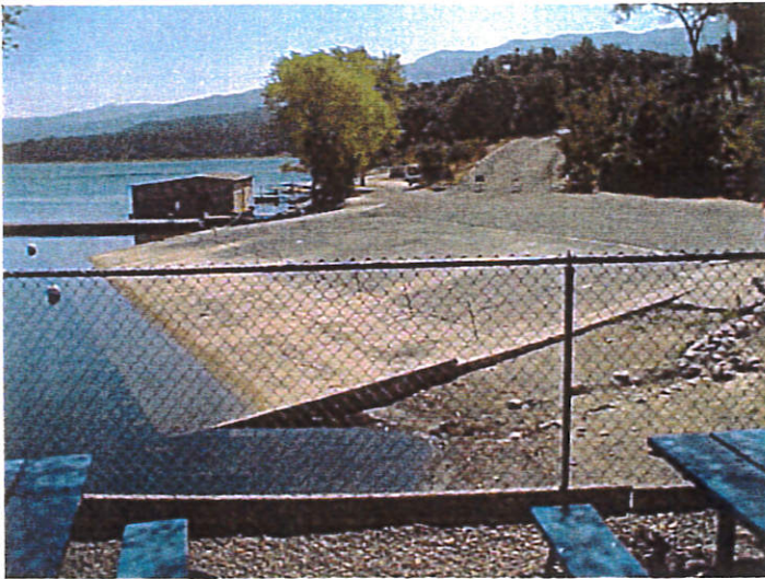
Launch Ramp looking West from Shops
