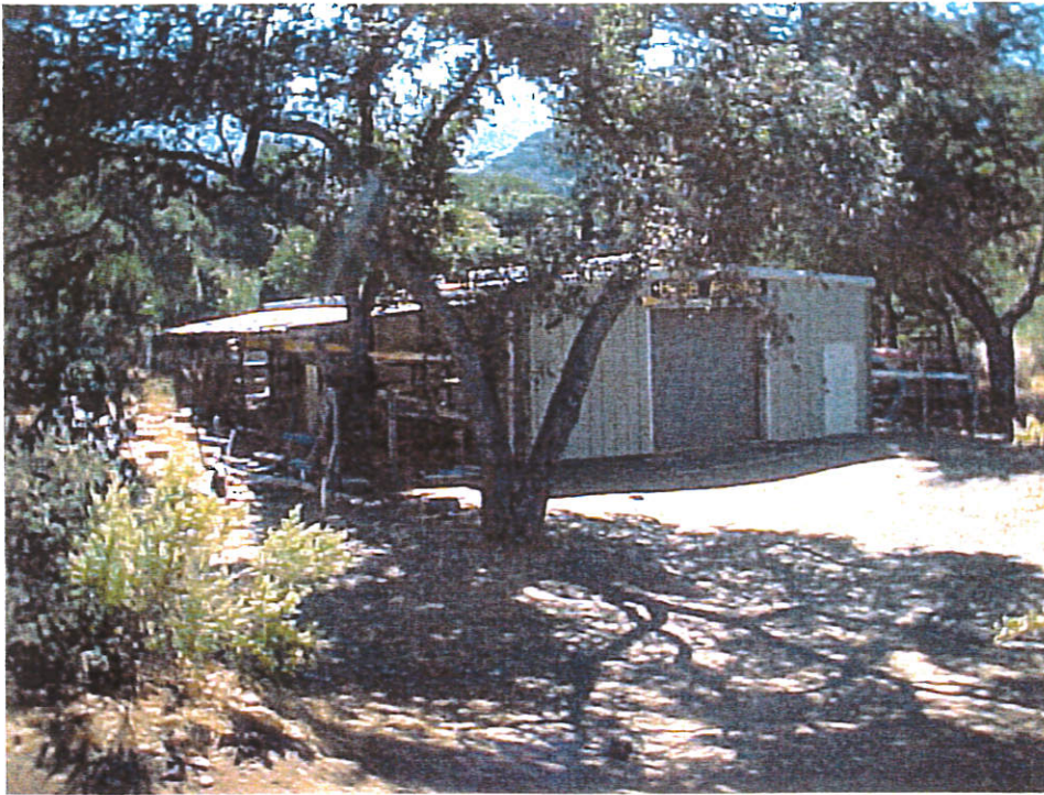
UCSB Crew Facilities looking South
