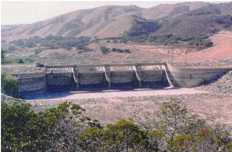
Upstream view of Bradbury Dam
