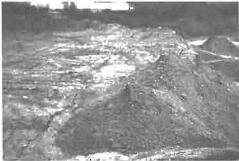
Cracks along crest of pile.
