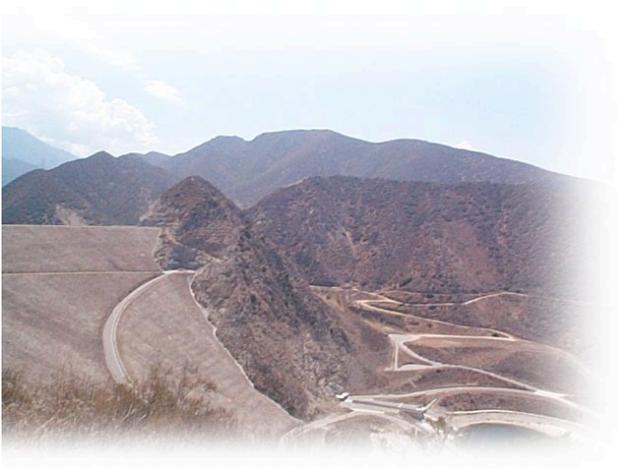
*Floodwaters slowed by Seven Oaks Dam (in the left of this picture) would be diverted at either the plunge pool (lower right of picture) or Cuttle Weir. New facilities would be built near the plunge pool, and captured water would be conveyed in new and existing facilities for use in the Muni and Western service areas.*
