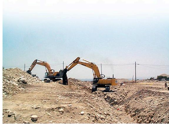
*Excavation in the Muni service area, such as the pipeline pictured here, can produce air quality impacts. During excavation and grading, fugitive dust emissions would be released, and construction equipment and vehicles would generate emissions.*
